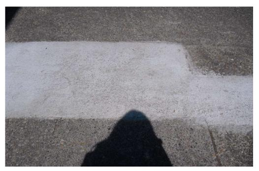
Photo 13. Sidewalk patching located along the southern property boundary.
