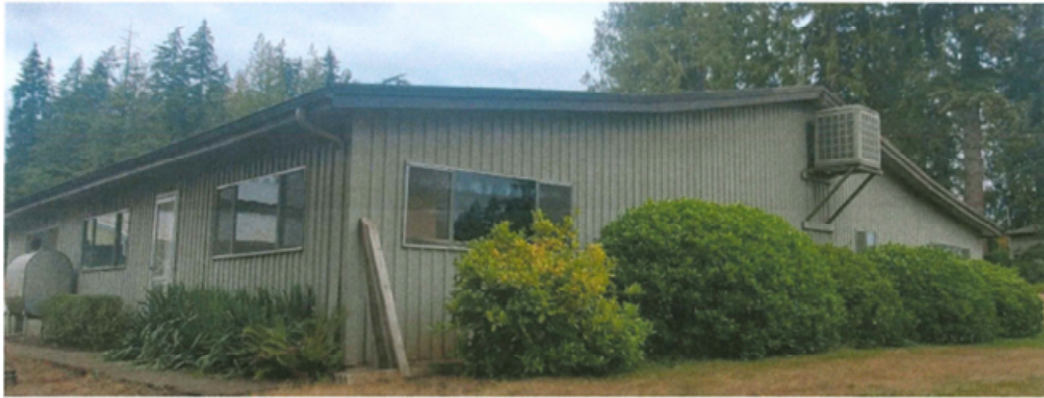
East and South views
