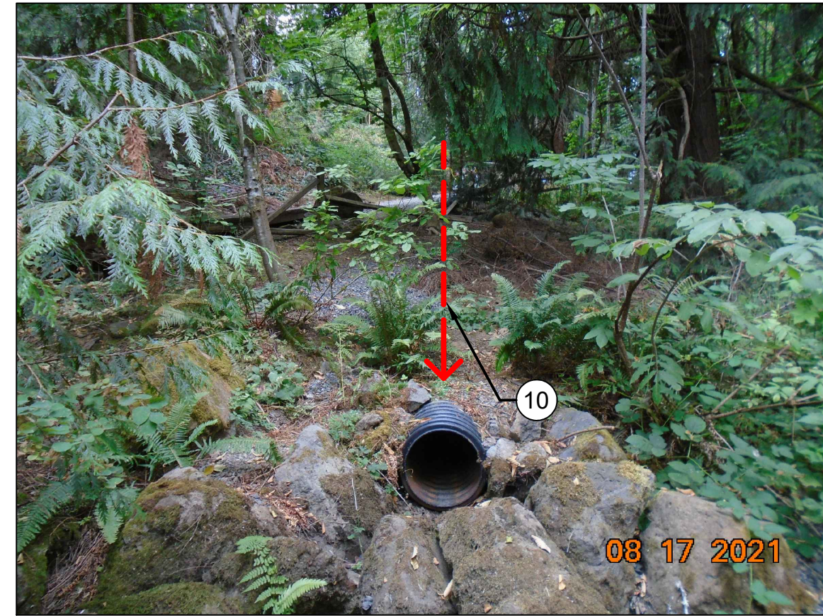
PHOTO 9 VIEW LOOKING NORTH FROM swDPT-00787 TO swCPT-00375
