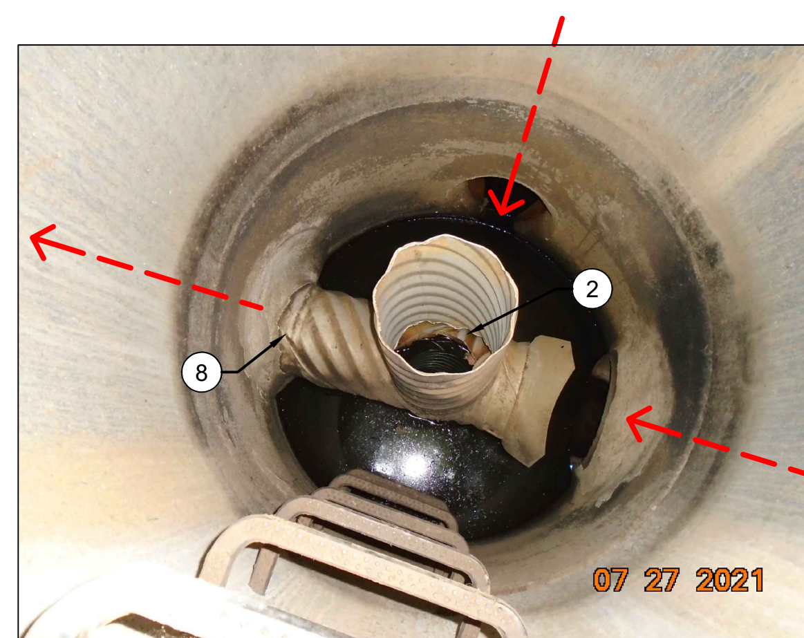
PHOTO 3 INTERIOR VIEW OF FLOW CONTROL TEE IN swCPT-00375
