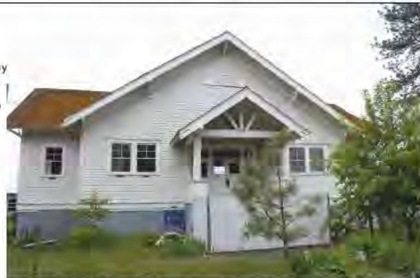
COURTESY PHOTO: CANBY SCHOOL DISTRICT - The Carus White Building is officially up for sale. It will either be moved by a buyer or it will be demolished.
