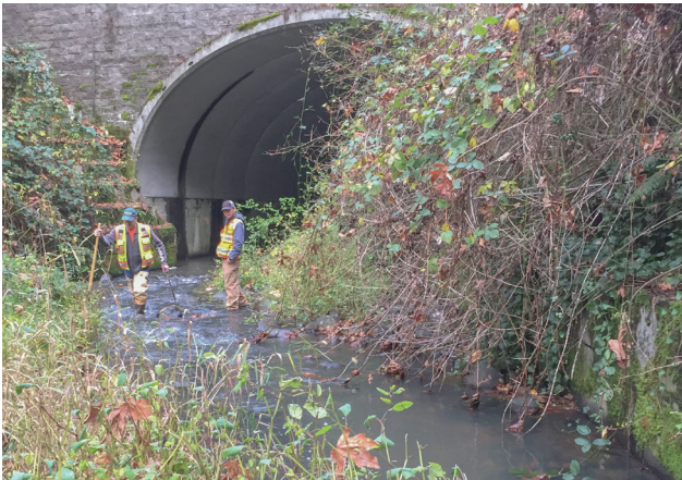
Staff inspect Foster Creek before bridge scour repairs to deflect flow away and preserve the retaining walls and culvert foundation at Baker's Ferry Road last year.
