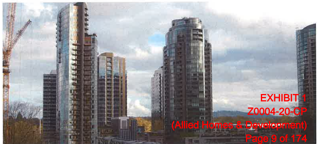
New Construction High-rise Condominiums Portland, Oregon
