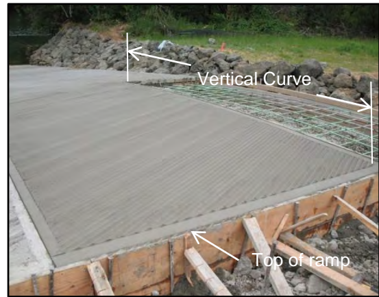
Photo 3-30 Vertical curve at top of launch ramp. Photo also shows block-out for float abutment.
