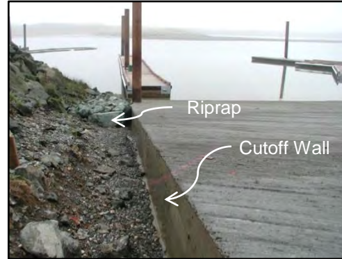
Photo 3-19 Cutoff wall along edge of ramp and riprap backfill
