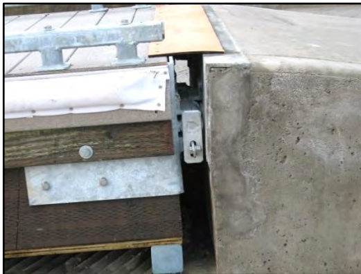
Photo 4-13 Hinged abutment connection
