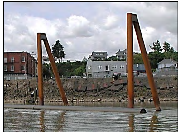
Photo 6-2 Batter supported vertical piles
