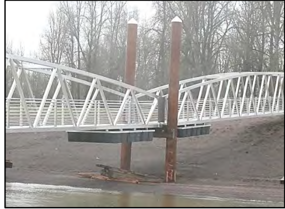
Photo 7-14 Pile supported connection for two gangways
