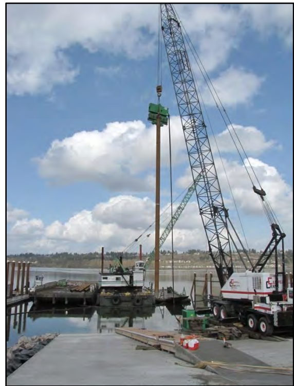
Photo 6-4 Land-based pile driving crane with vibratory hammer
