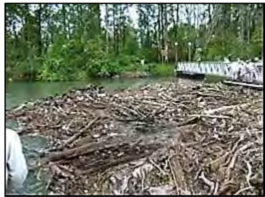
Photo 8-2 Debris accumulation at a transient float facility. This occurred during a normal high water event. A debris deflection boom was subsequently installed to protect the facility.
