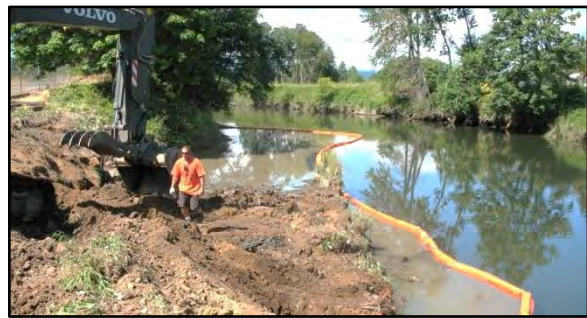
Photo 3-27 Floating silt curtain in-place to isolate work area and control turbidity
