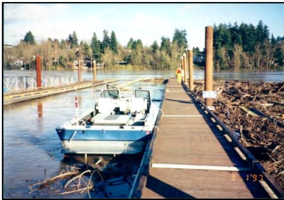
Photo 8-1 Debris at launch ramp floats. Boarding floats are not generally susceptible to debris of this magnitude but this occurred during a 100-year flood event.
