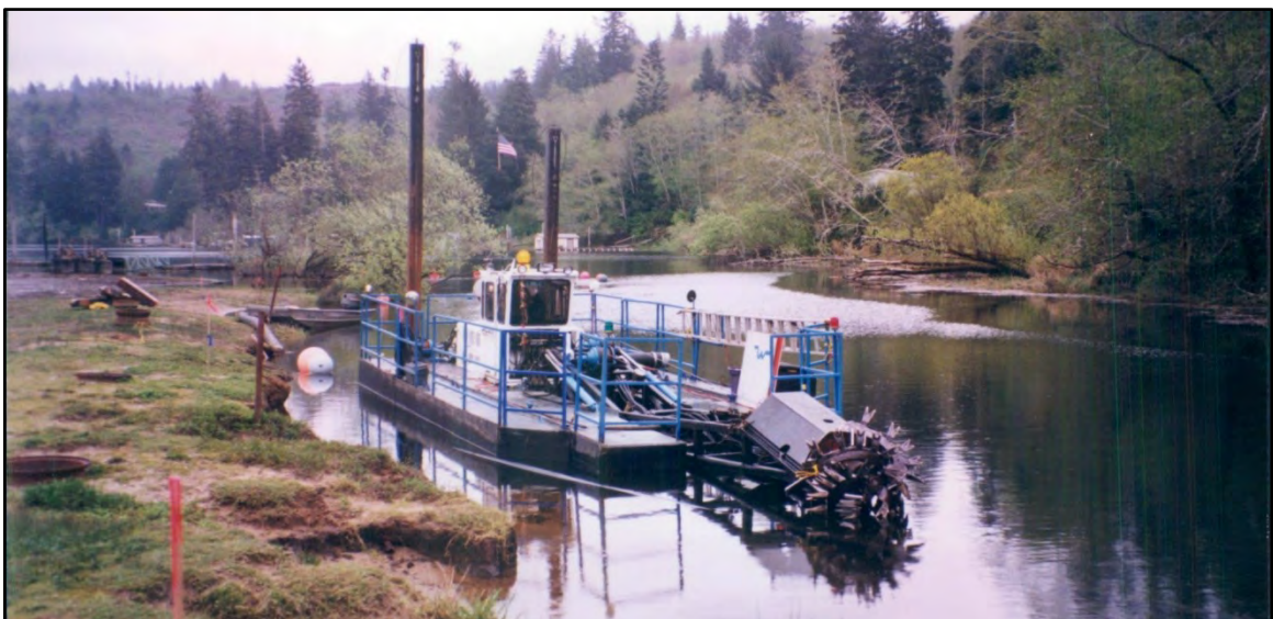
Photo 2-3 Suction dredging barge
