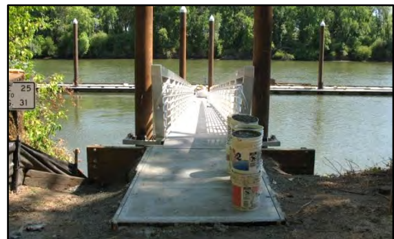
Photo 7-12 Timber bulkhead connection
