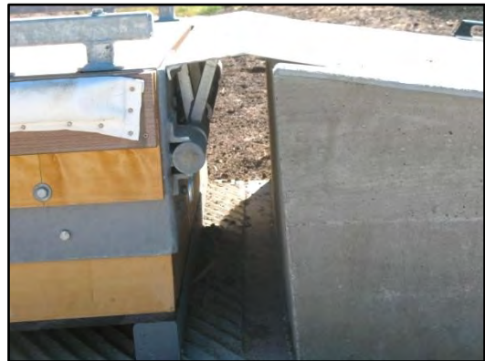
Photo 4-14 Transition plate connection
