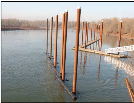
Photo 8-4 Poly-pipe debris boom
