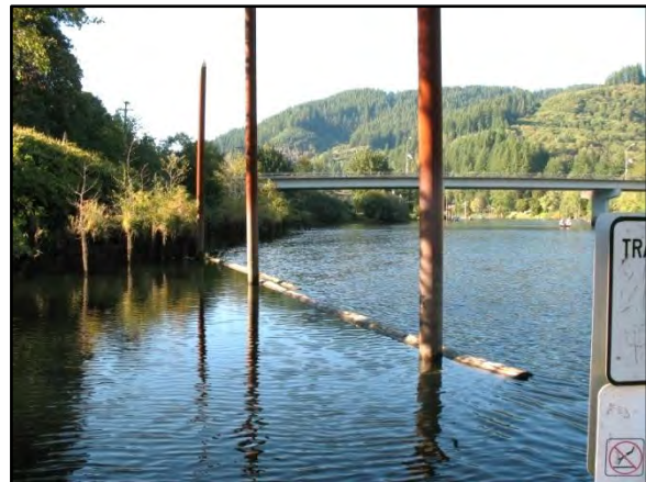
Photo 8-3 Log debris boom
