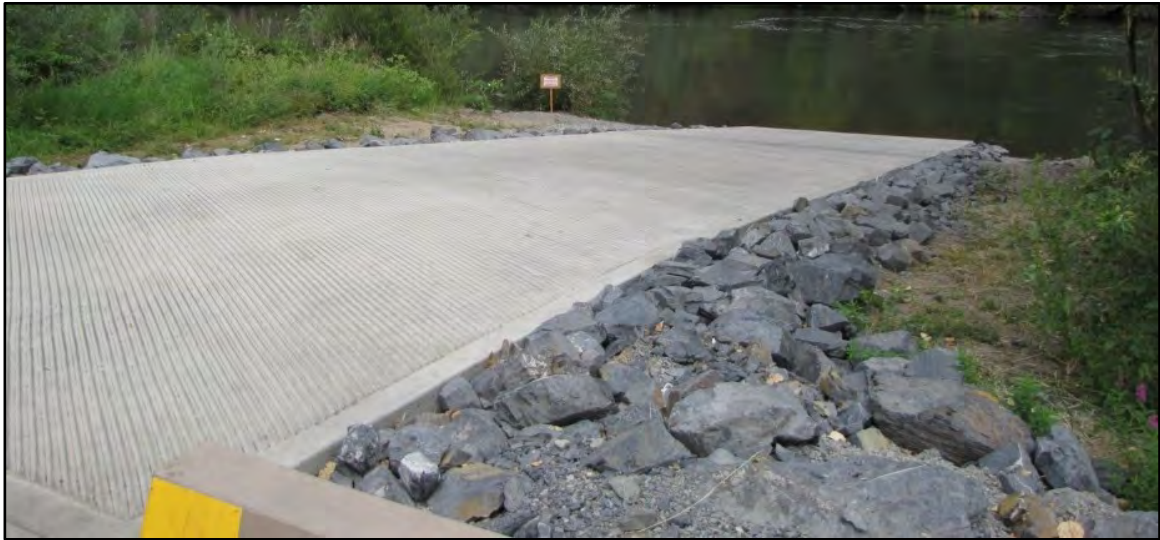
Photo 3-9 Single-lane launch ramp without boarding floats
