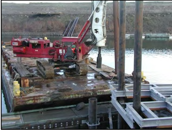
Photo 6-7 Drill rig preparing for drilling
