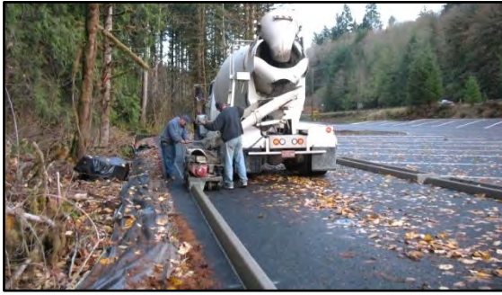
Photo 9-4 Installation of extruded concrete curb
