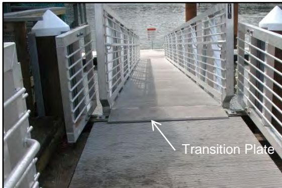
Photo 7-4 Transition plate at shore-end of gangway
