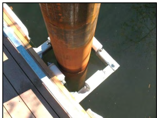
Photo 4-12 External pile hoop
