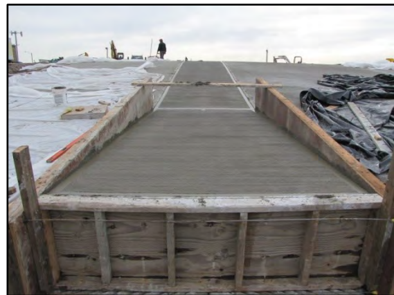
Photo 4-6 Float abutment and walkway after placement of concrete. Both have a broom finish.
