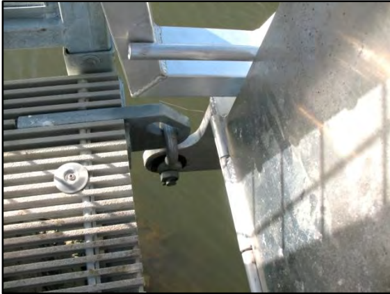
Photo 7-6 Link connection at pier-end of gangway
