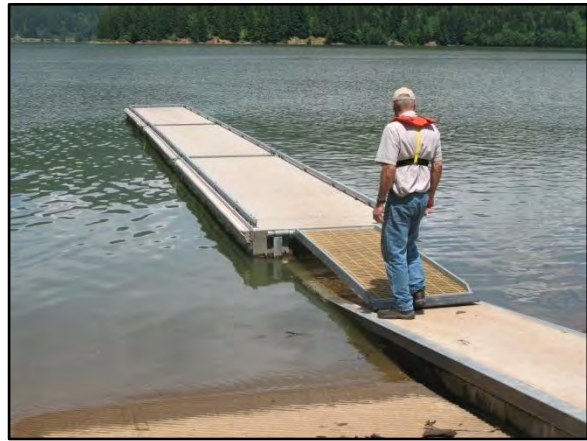
Photo 4-8 Self-adjusting boarding floats
