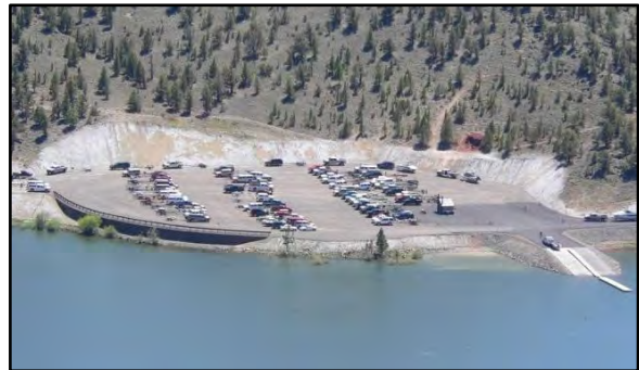
Photo 3-1 Launch facility where a large cut (parking lot) and fill (launch ramp) was required to fit the local topography
