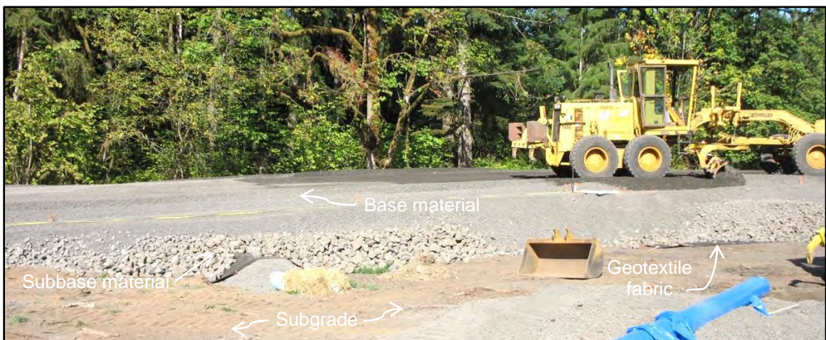
Photo 9-3 Pavement section during final grading
