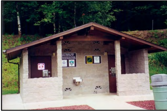
Photo 10-6 Site-built flush restroom
