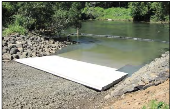
Photo 3-24 Proper number of precast planks above the water line for transition to cast-in-place ramp
