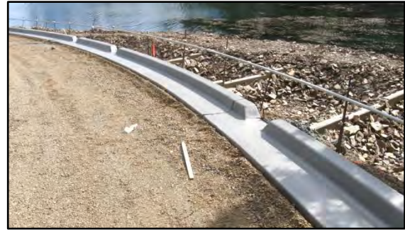
Photo 9-5 Installation of cast-in-place concrete curb with curb cuts for sheet drainage
