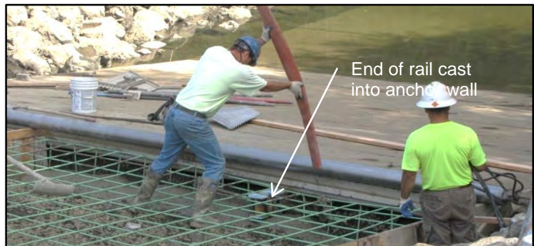
Photo 3-29 Transition from precast planks to cast-in-place concrete. This photo shows the 24" deep anchor wall being poured. A rebar pin through the web of the rail and rebar hooks into the anchor wall tie the precast planks and rail system to the cast-in-place launch ramp.
