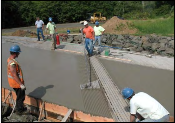
Photo 3-32 Cutting grooves into fresh concrete. The plank acts as a guide for groove alignment and tool control.
