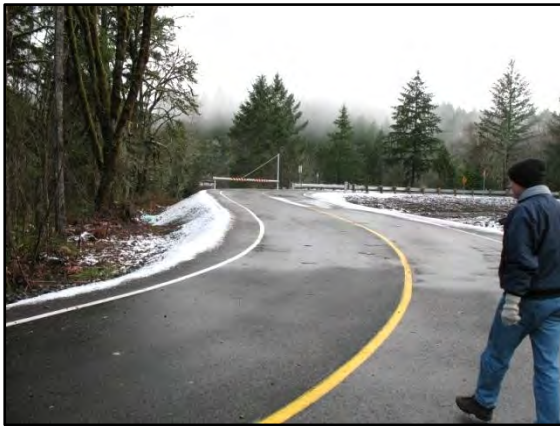
Photo 9-6 Typical two-lane access road
