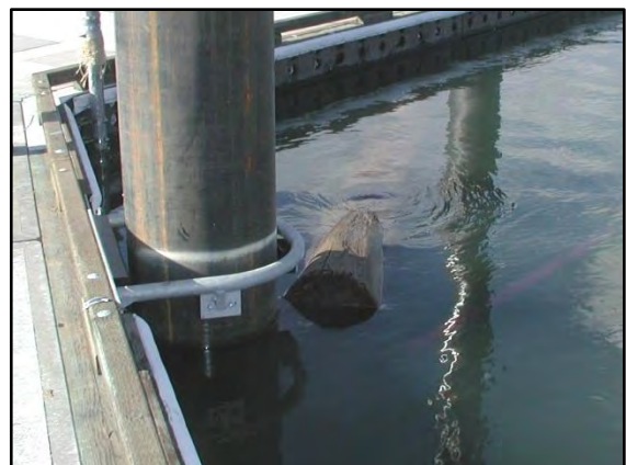
Photo 5-14 External pile hoop
