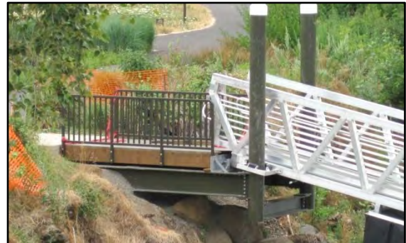
Photo 7-10 Cantilevered steel and timber fixed-pier connection
