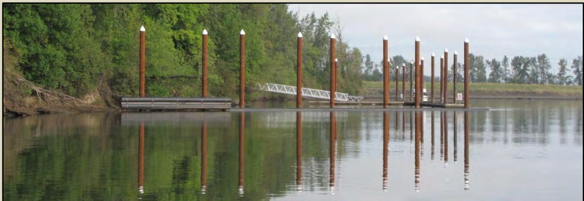
Photo 8-7 Poly-pipe debris boom protecting a transient facility
