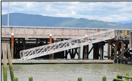
Photo 7-9 Timber fixed-pier connection
