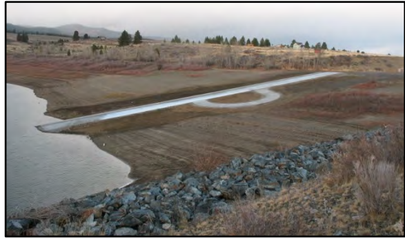
Photo 3-8 This launch ramp is nearly 400 feet in length and is designed with a turnout at the halfway point
