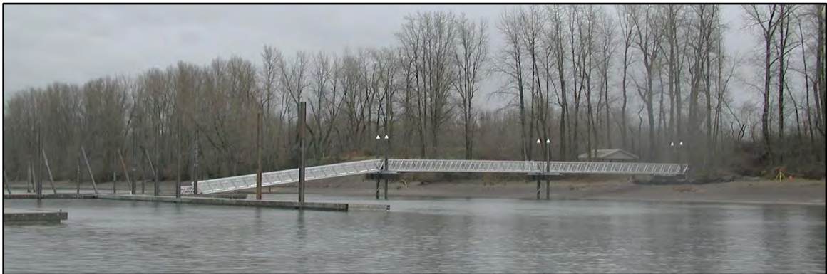
Photo 7-2 A series of gangways is required at this facility to access the transient floats. The two shoreward gangways are considered elevated walkways.
