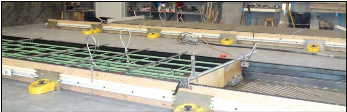
Photo 3-22 Shop fabricated precast planks. The form in the foreground is ready for placement of concrete. The form in the background has concrete in place. These planks are cast upside. The cable loops are used to lift and turn the planks and will be cut off flush with the bottom.
