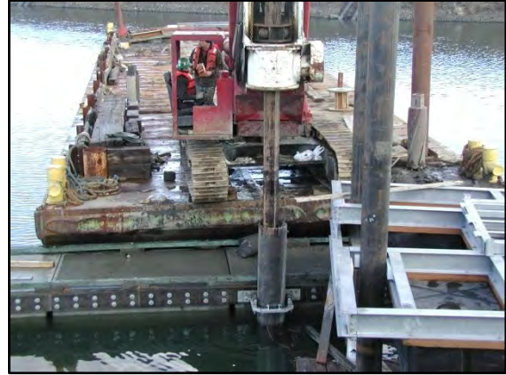
Photo 6-8 Drill rig in position and drilling
