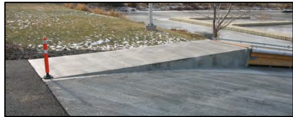
Photo 4-4 Concrete float abutment
