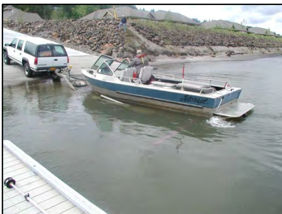
Photo 3-5 Proper ramp slope keeps tow vehicle out of the water and provides access to the trailer
