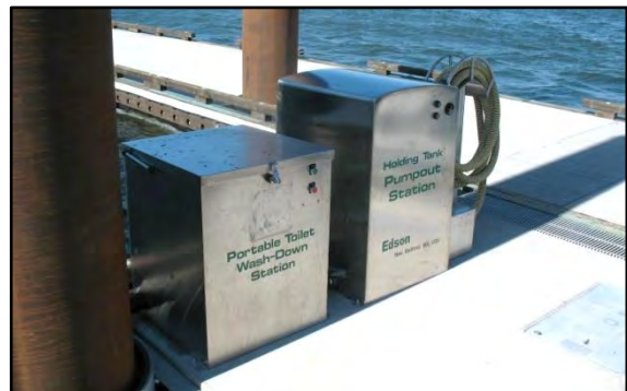
Photo 5-2 Float mounted pumpout and dump station
