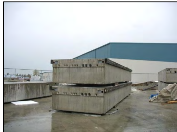
Photo 5-8 Individual float sections connected together with wood walers to make sub-assemblies. The holes in the end of the float are utility chases.
