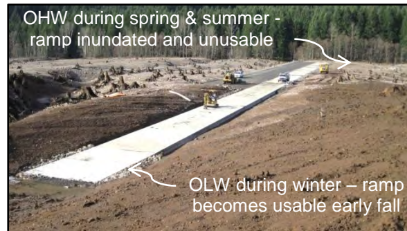
Photo 3-7 Low water launch ramp at a reservoir
