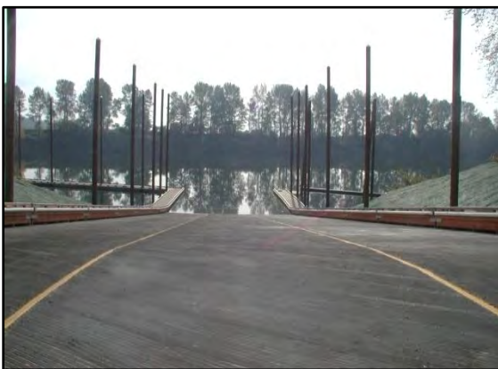
Photo 3-13 Three-lane launch ramp with boarding floats down both sides
