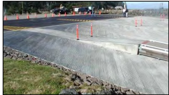
Photo 3-35 Broom finish on walkway leading to float abutment
