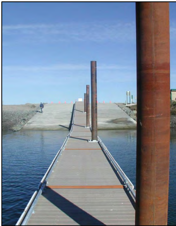
Photo 3-11 Two-lane launch ramp with boarding floats down the center between lanes
