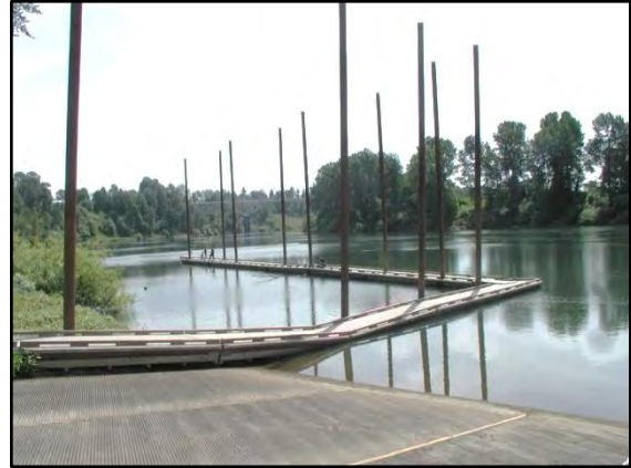
Photo 5-16 Boarding float connection to uplands
