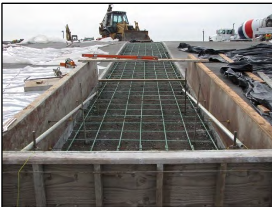
Photo 4-5 Float abutment formed and ready for concrete
