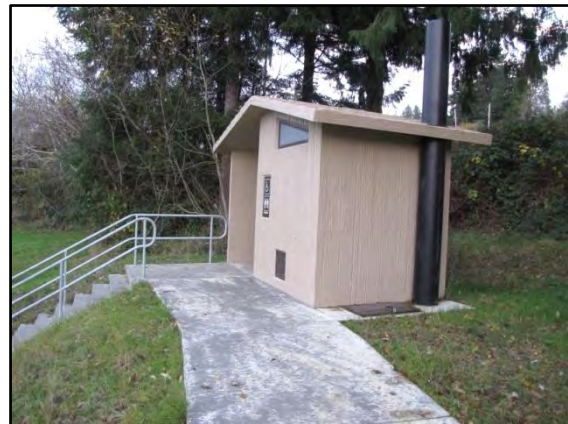
Photo 10-9 Precast concrete vault toilet
