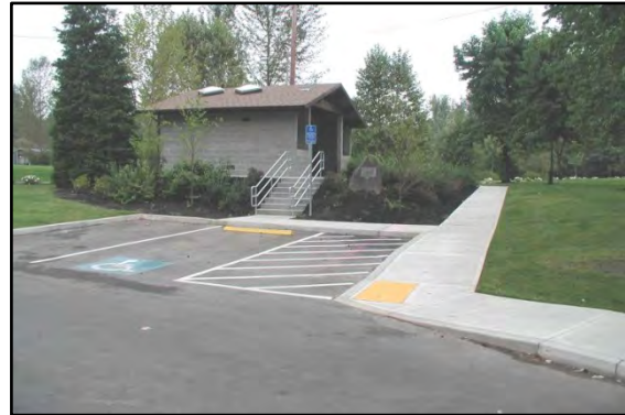
Photo 10-3 Restroom built on fill to be above the 100-yr flood elevation. The sidewalk provides ADA accessibility while the stairs provide a more direct route.
