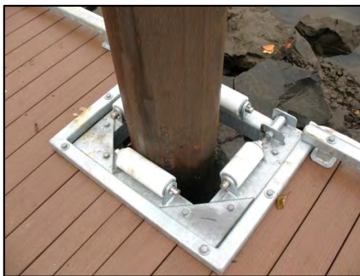
Photo 4-11 Internal pile pocket
