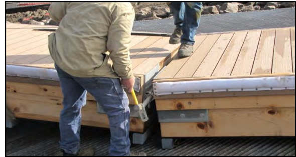
Photo 4-15 Connecting boarding float sections
