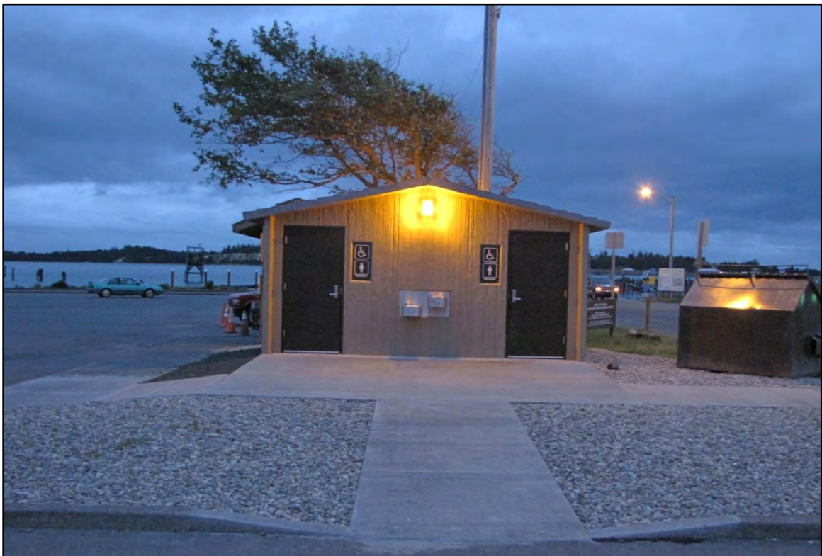
Photo 11-1 This restroom incorporates two drinking fountains (one ADA compliant) and exterior lighting. The pole light in the background is located at the top of the launch ramp.
