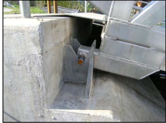
Photo 7-7 Lift-off connection at abutment end of gangway
