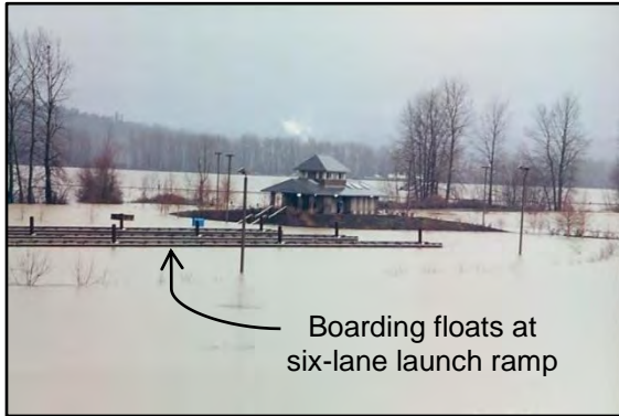
Photo 10-2 This photo was taken during a 100-yr flood event. The restroom was built well above the flood elevation.
