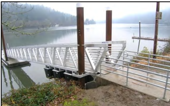
Photo 7-11 Concrete abutment connection
