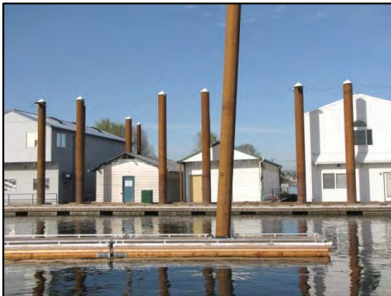
Photo 6-1 Battered boarding float pile in foreground and vertical transient float piles in background
