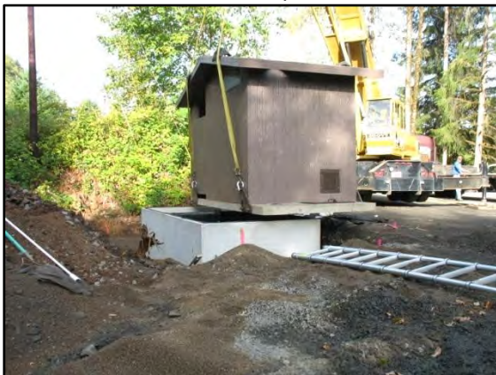
Photo 10-8 Installation of precast vault toilet
