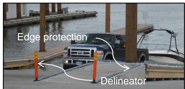
Photo 4-7 Traffic delineators and edge protection
