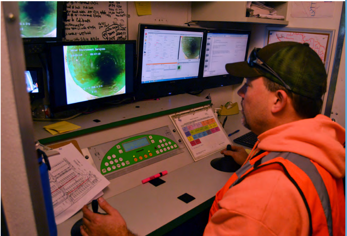
WES field operators using video to inspect the pipes
