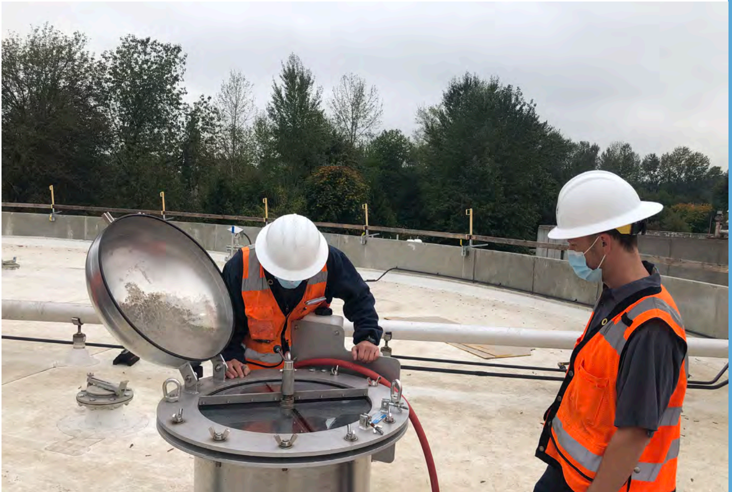
Operators look through the new digester view port to verify mixing
