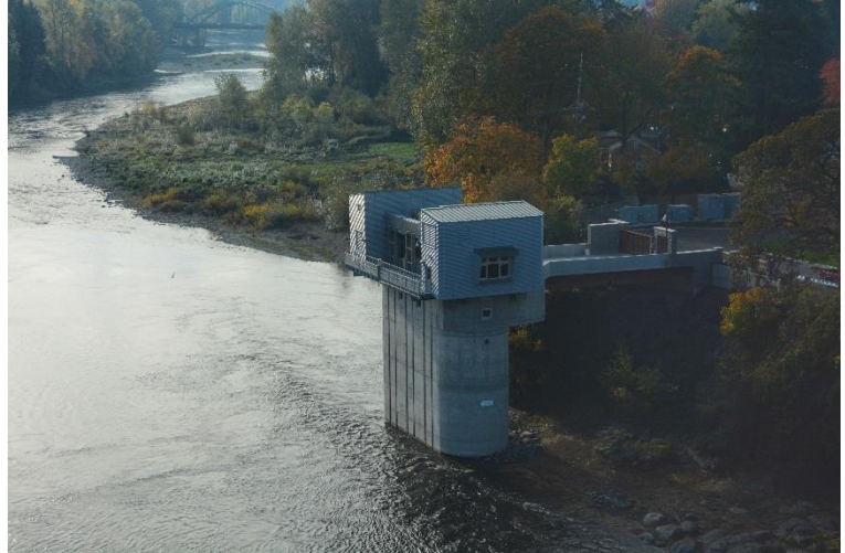
Lake Oswego Tigard Raw Water Intake
