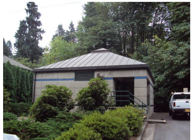
WES Telemetry System Replacement
