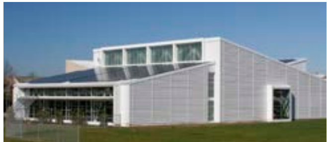
Solar PV: E Portland Community Center Aquatics Addition
