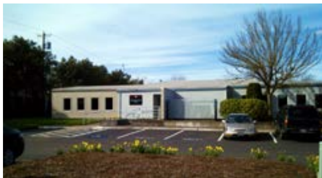
Existing screening of equipment at Technology Services annex (former Assessment and Tax Facility) Fence: Painted wood slats, 8-foot tall.
