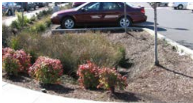
Parking Lot Bioswale
