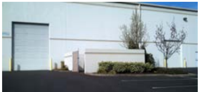
Garbage enclosure at Silver Oak Fence: Slatted chain link and concrete, 6-foot high.
