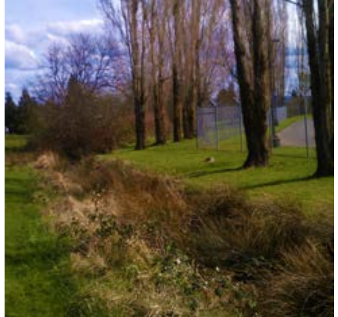
Existing perimeter fence, ADF. Mud Creek Wetland foreground Fence: Chain link with barbed wire, 8-foot high.
