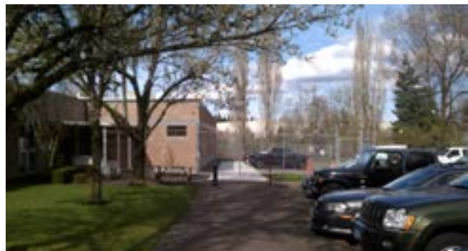
New medical wing addition at ADF Fence: Chain link with barbed wire, 8-foot high.
