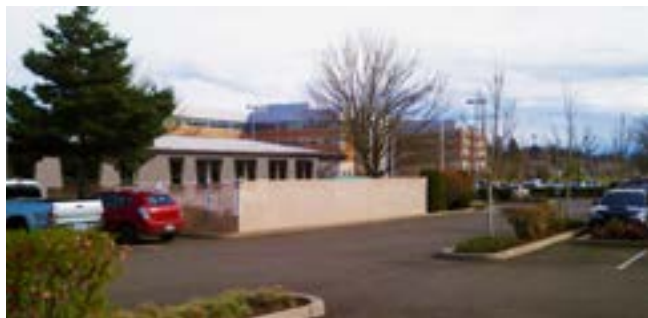
Existing screening of equipment at Technology Services Fence: Slatted chain link, 4-foot high.
