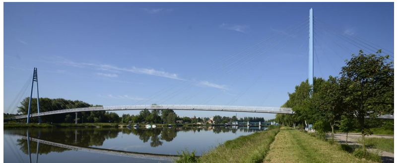
Pedestrian Bridge across the Elbe River, Celakovice, Czech Republic
