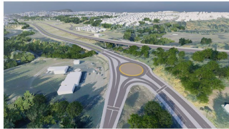
Rock Creek Junction will be converted into multi-lane roundabout to improve safety and provide adequate capacity following the development of the Sunrise Gateway Corridor.
