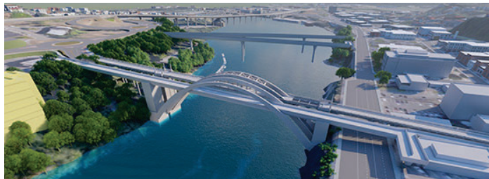
Oregon City – West Linn Pedestrian - Bicycle Bridge Concept Plan: Rendering to convey concepts and address concerns about viewsheds and historical impacts. ( See animation )
