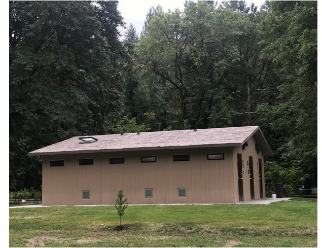
New Restroom Structure
