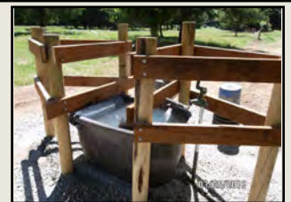
Livestock water system
