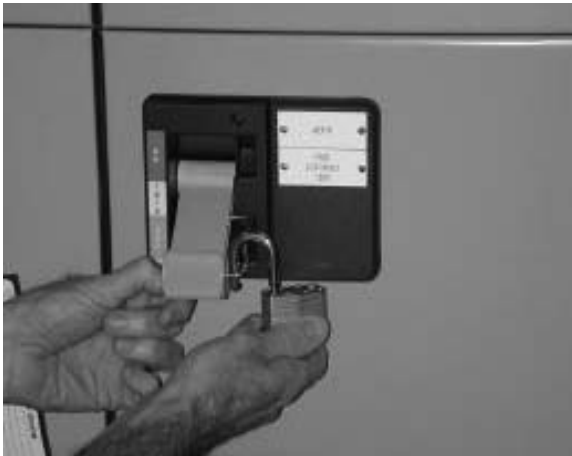
Figure 36. Locking Out a Disconnect
