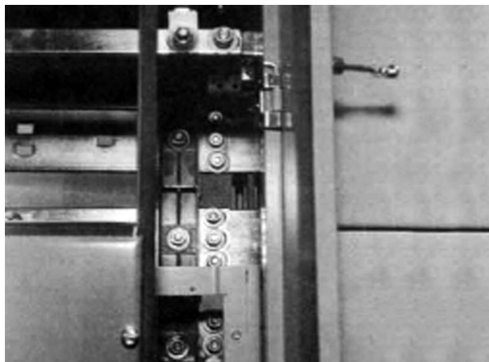
Figure 5. Access to Left-Hand Splice Plate Connections
