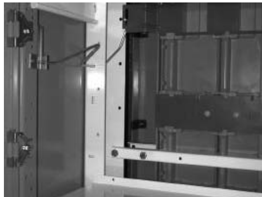
Figure 33. Shutter Arm Linkage
