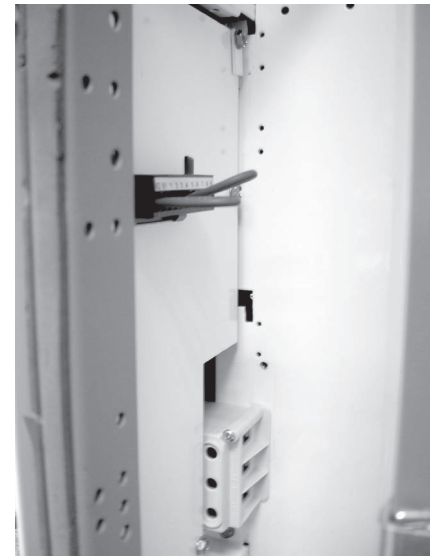
Figure 15a. Pull-Apart Terminal Blocks
