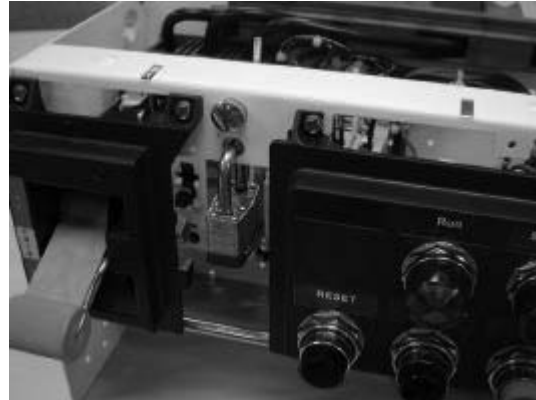
Figure 31. Unit Locked in Detent Position
