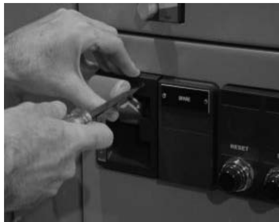
Figure 35. Defeater Mechanism
