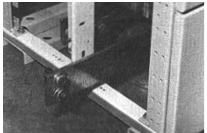
Figure 14. Splice Plate Attached to Freedom FlashGard Neutral Bus
