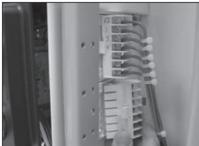
Figure 29. Disengaging Pull-Apart Terminal Blocks
