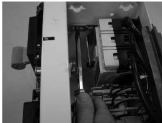
Figure 32. Operating Handle Linkage Adjustment
