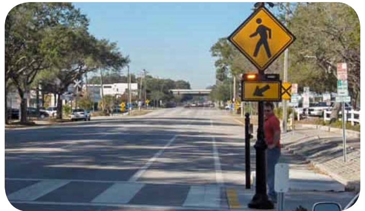
Signalized pedestrian crossing
