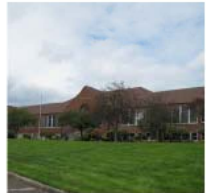
Concord Elementary School
