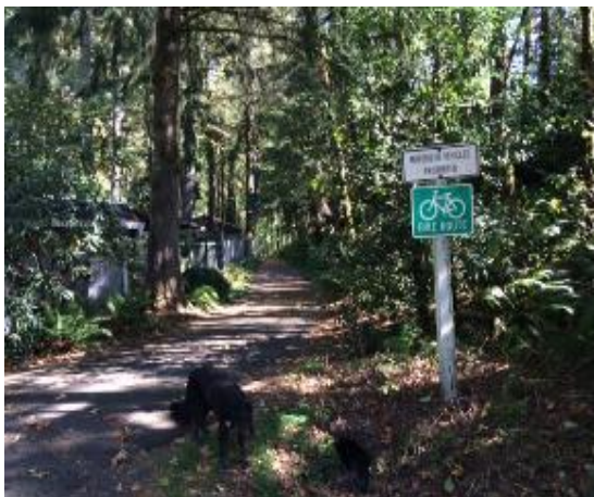
Figure 10: Entrance to the US 26 underpass for bicycle riders and pedestrians
