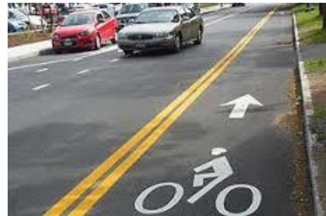
Figure 21: Example of a contraflow bike lane that allows bicycle riders to ride in the opposite direction of vehicular traffic
