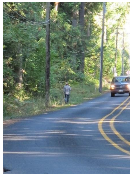
Figure 16: Existing walking conditions on Welches Road
