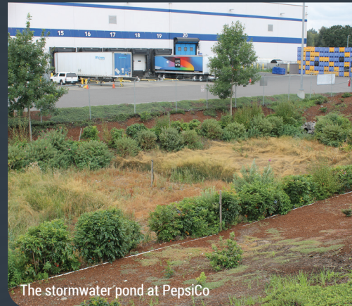
Inspecting a stormwater facility
