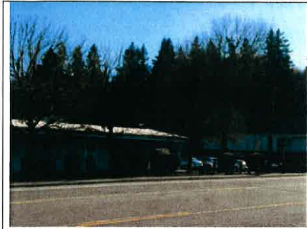
Looking south to subject's property line and parking.
