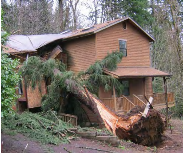
Windstorm damage – March 13, 2011 Source: Clackamas County Disaster Management
