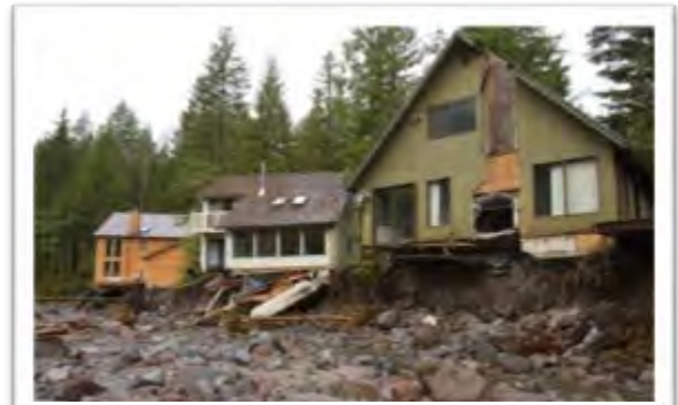
Sandy River Channel Migration Damage January 16, 2011 Source: Oregonian
