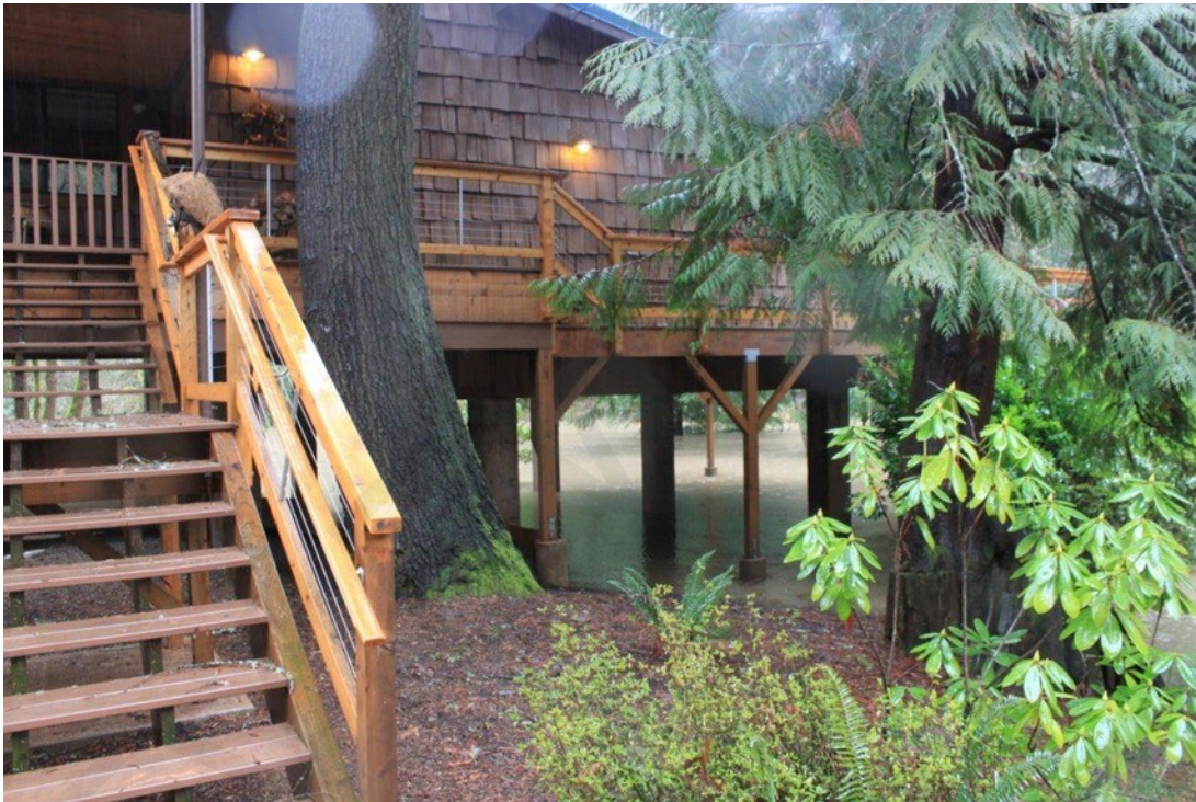
Mitigation Success - Abernethy Creek elevation completed in March 2010 and successfully tested on January 19, 2012. Source: Clackamas County
