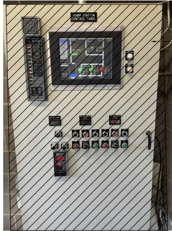
REMOVE EXISTING CONTROL PANEL AND INSTALL NEW CONTROL PANEL IN SAME LOCATION. SALVAGE CONTROL PANEL AND PROVIDE TO WATER ENVIRONMENT SERVICES FOR SPARE PARTS.
