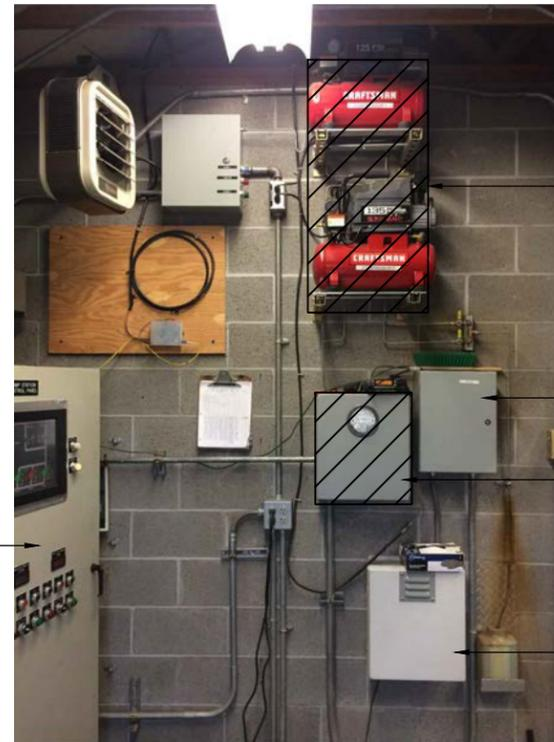
REMOVE EXISTING BUBBLER SYSTEM COMPRESSORS DELIVER REMOVED COMPRESSORS TO WES.
