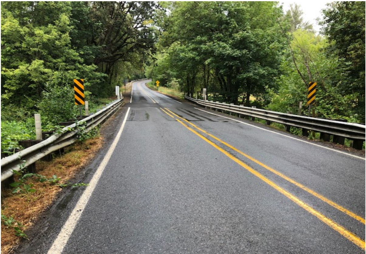
Exhibit 2-1: Existing Bridge Site looking North on Canby Marquam Highway
