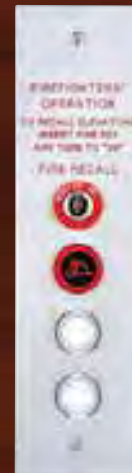
Intermediate hall station With fire services devices
