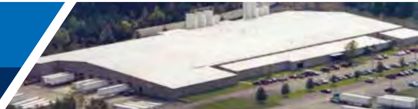
JM TPO manufacturing facility in Scottsboro, AL
