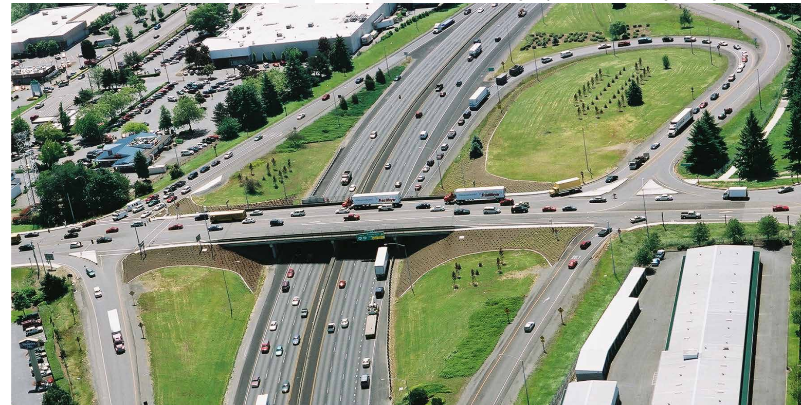
Highway 212/I-205 Interchange looking south
