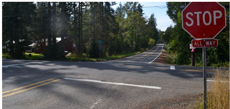
Example of roadway without shoulders (SE Tillstrom Road at SE 222 nd Avenue)
