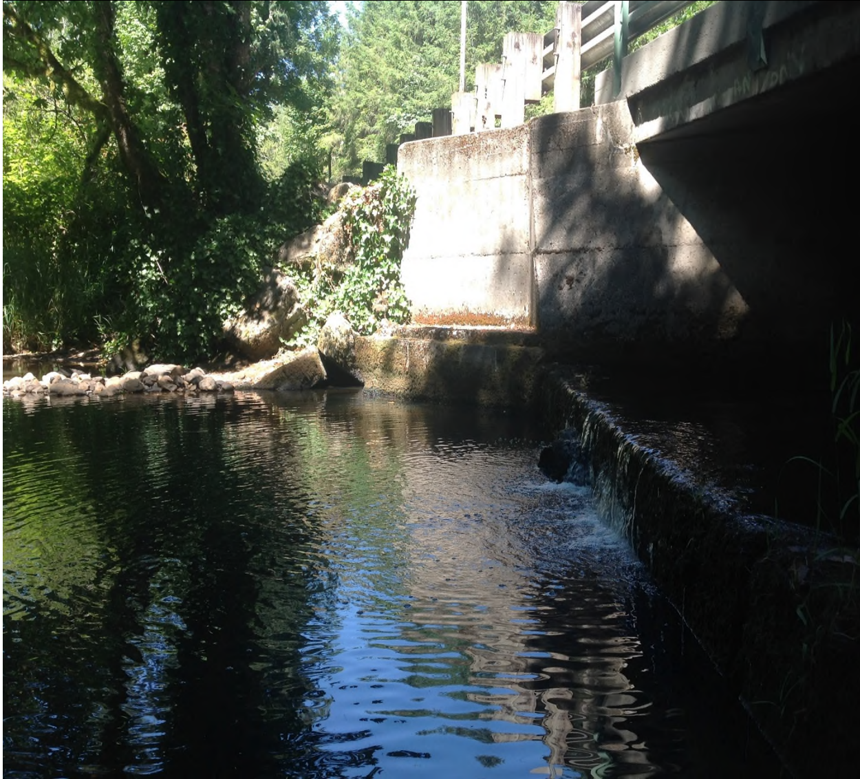
Photo 1 Looking: Left bank to right bank Note: Perched, concrete floor
