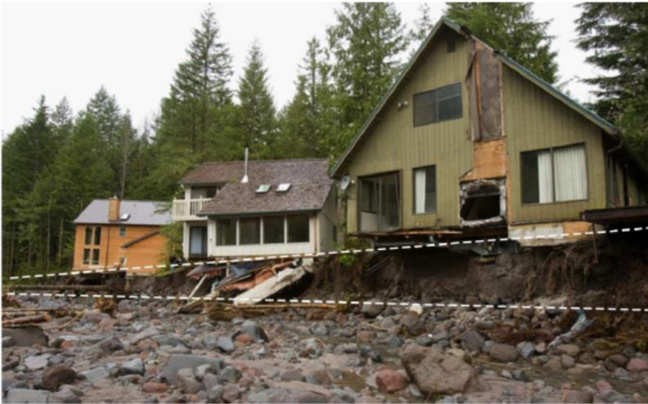
Damages resulting from January 16, 2011 flood, Zig Zag Village, Upper Sandy River
