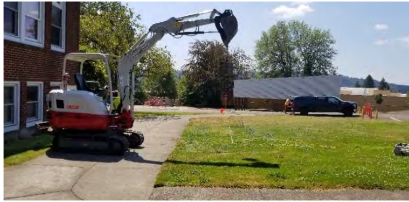
Photo 1. Seismic Refraction using 300 # weight drop.
