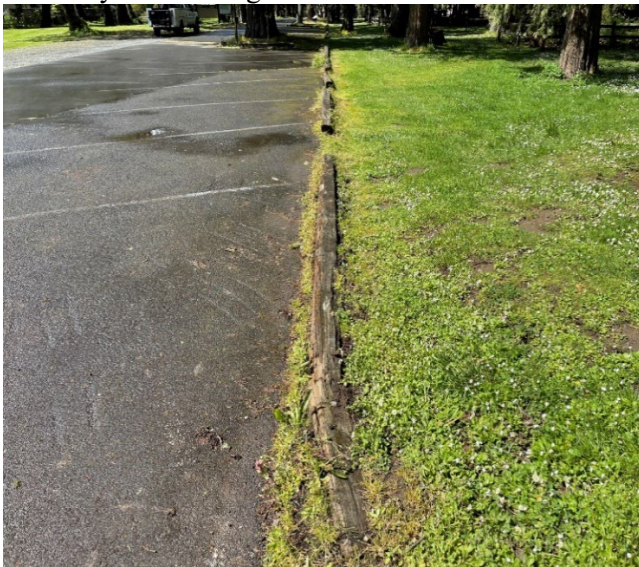
Existing wheel stop and parking view
