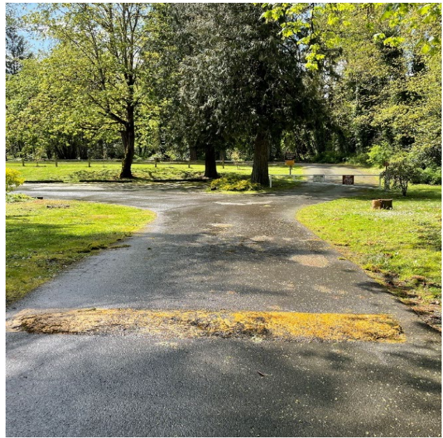
Existing roadway and speed humps
