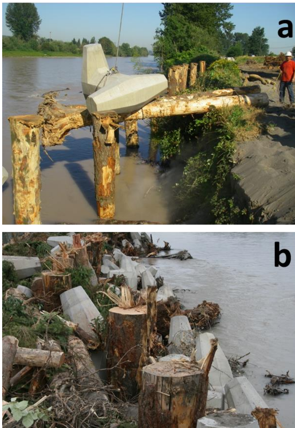
Figure 44A/B. Using a combination of timber and dolosse has been used in Washington State as a more restorative alternative to traditional measures to protect levees and roads. The dolosse are eight ton unreinforced concrete jacks that provide a complex interlocking shape emulating the function of natural snags. The top photo (a) shows how a dolo and attached log can be easily lowered into place and avoid expensive dewatering. Using the dolosse with logs creates a complex structure as shown in bottom photo (b) that can settle if undercut by scour, but without the need of rock or cable. The structures can be designed with lots of wood so the dolosse aren't even visible. Since they are self-settling, these structures don't need to be deeply excavated into the river bed as rock revetments or ELJs constructed only using timber (Figure 42, 43). Photos are of complex revetment built to protect a levee along the Lower Puyallup River in Fife, WA.
