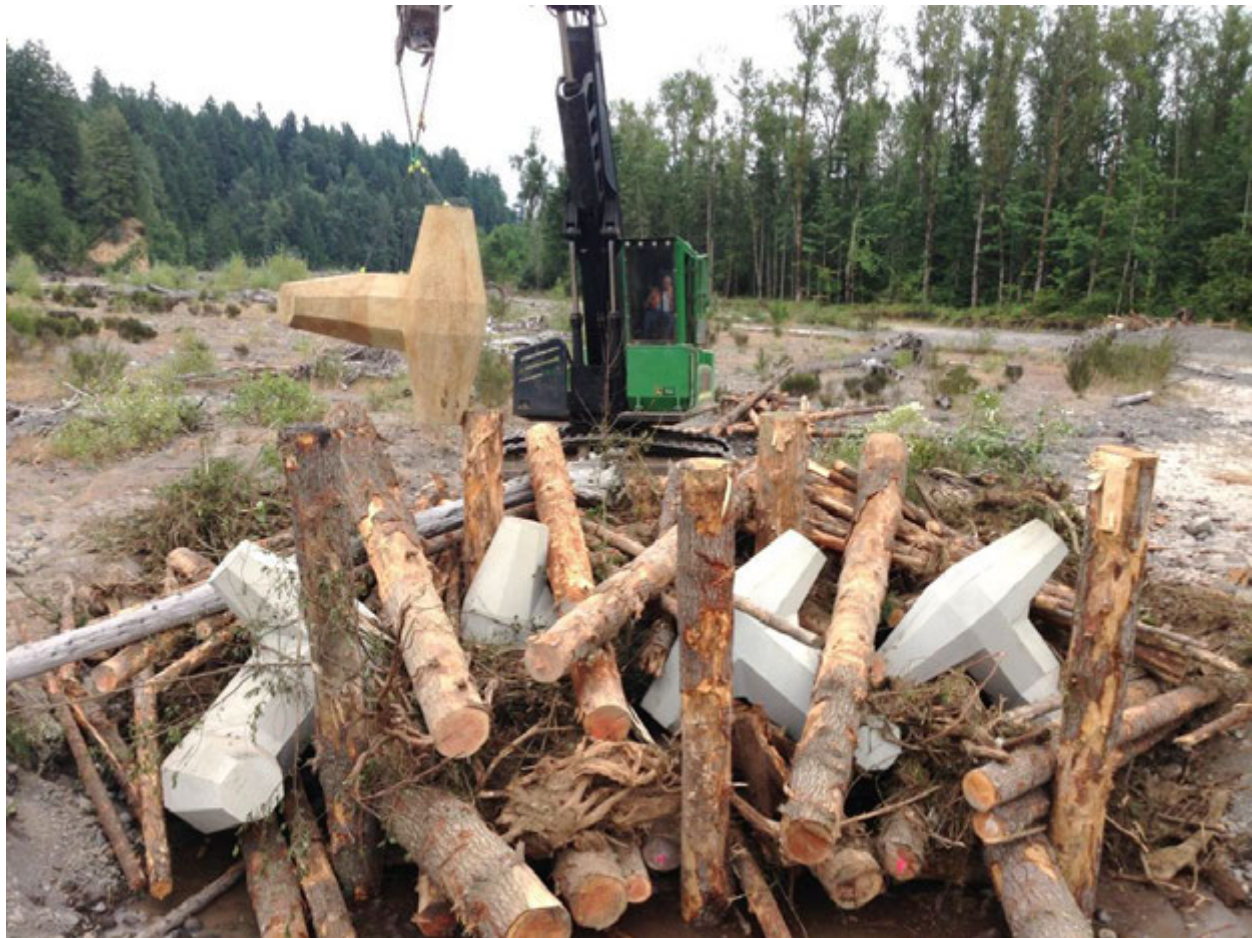
Figure 45. Construction of ELJ using 8 ton dolosse in Upper Puyallup (same structures depicted in Figure 40). The dolosse offer an interlocking ballast the structure can settle into river bed if undermined without coming apart. This means the structures don't require as much excavation, lowering construction impacts and costs. Dolosse are covered with alluvium and wood so they are barely visible in completed structure. View is looking upstream into core of the structure.
