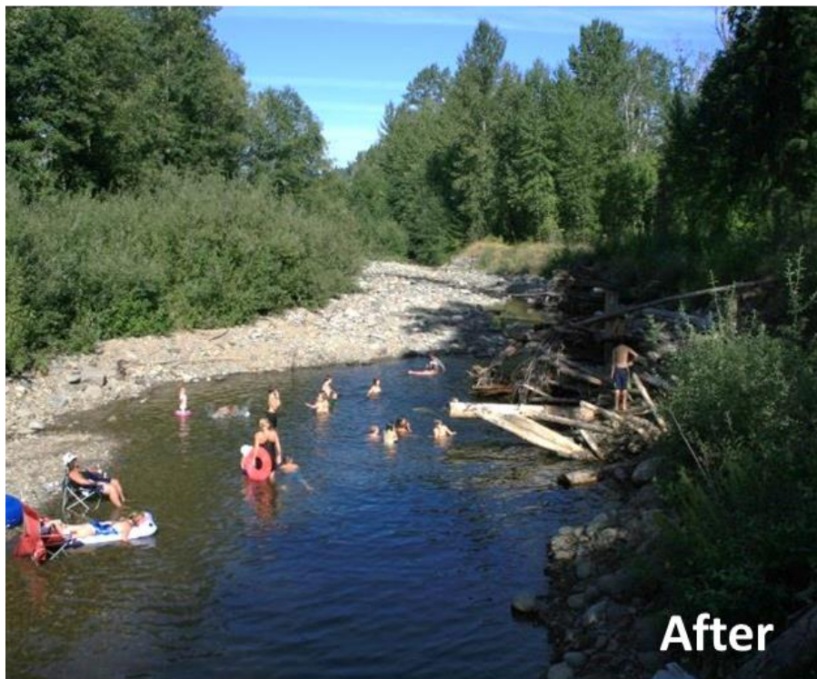
Figure 47. Illustration of how river restoration doesn't just benefit salmon, but also people. The photos above are looking upstream at same site before and after restoration of the Mashel River in Eatonville, WA. In 2006 a rock revetment was replaced by a series of engineered logjams. The logjams formed deep pools where none had previously existed and created greater textural variance in the channel. Over 400 juvenile salmon were documented in each of the ELJ pools and during the summer the pools became popular swimming holes for Eatonville residents.
