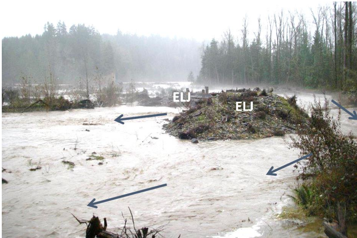
Figure 42. The Upper Puyallup project during high flow in 2014 looking upstream at two of engineered logjams (ELJs) in the energy dissipation area (side channel zone). View is from complex timber revetment on Upper Puyallup River's left bank. The ELJs are splitting flow into smaller channels before the flow reaches the bank. The ELJ is one of six forming an array of structures to keep the main channel from approaching the bank. Photo by Tom Nelson.
