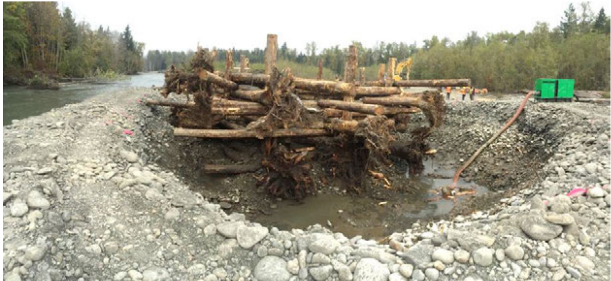
Figure 43. Example of engineered logjam that doesn't have self-settling elements of previous examples. This structure is deeply embedded into the river so that it can withstand scour without being compromised. Note people on right side of the structure. Pit is 16 feet deep and timber posts extend deeper. Elwha River 2014.
