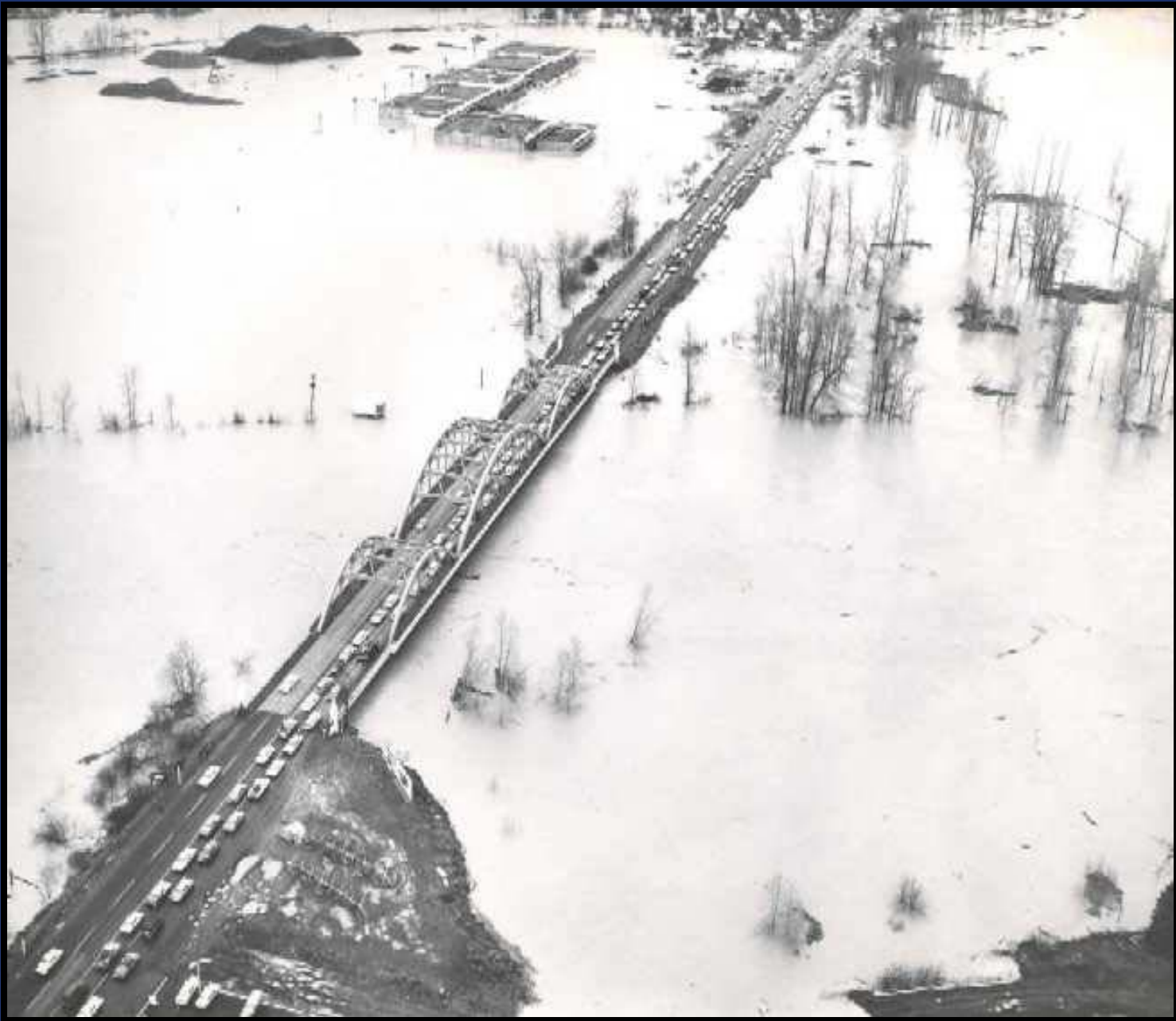
December 1964 Flood - Hwy 99E Clackamas River Bridge
