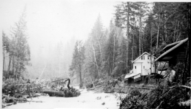
Damage to summer homes on private lands, Zigzag area.
