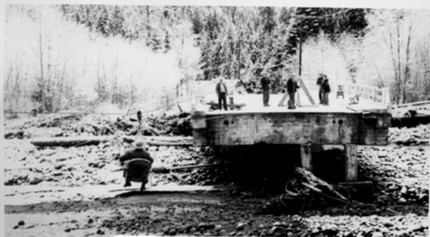
Emergency crossing of Zigzag River on Highway 26 bridge.
