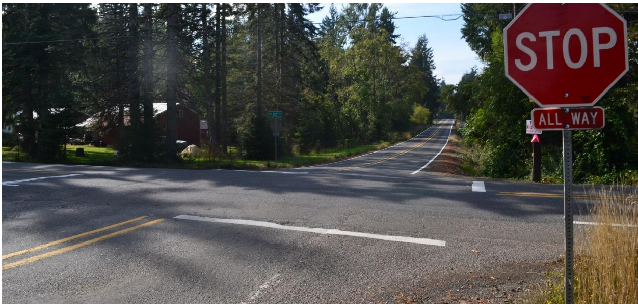
Exhibit 7. SE Tillstrom Road (Located at SE 222 nd Avenue) with No Shoulders
