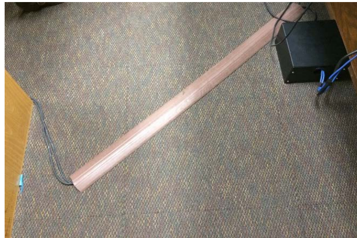
Cables at litigation well in courtroom
