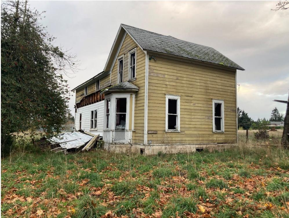
*House today (showing broken windows, exposed foundation and collapsed porch blocking the front door)*
