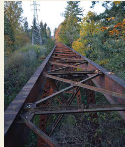
Eagle Creek Trestle
