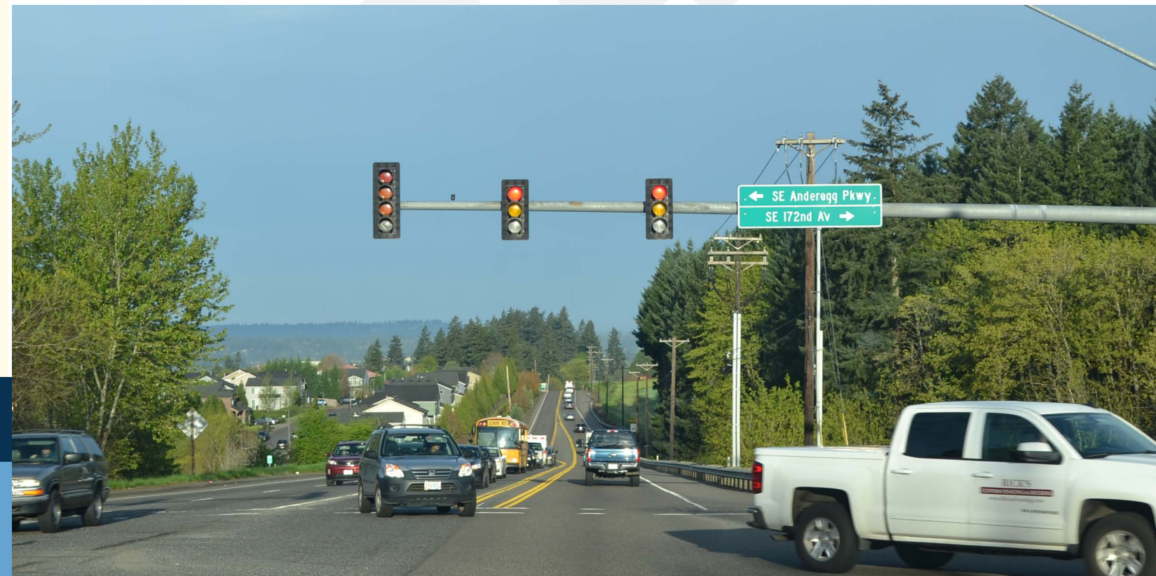
SE 172nd Avenue/Highway 212 looking west
