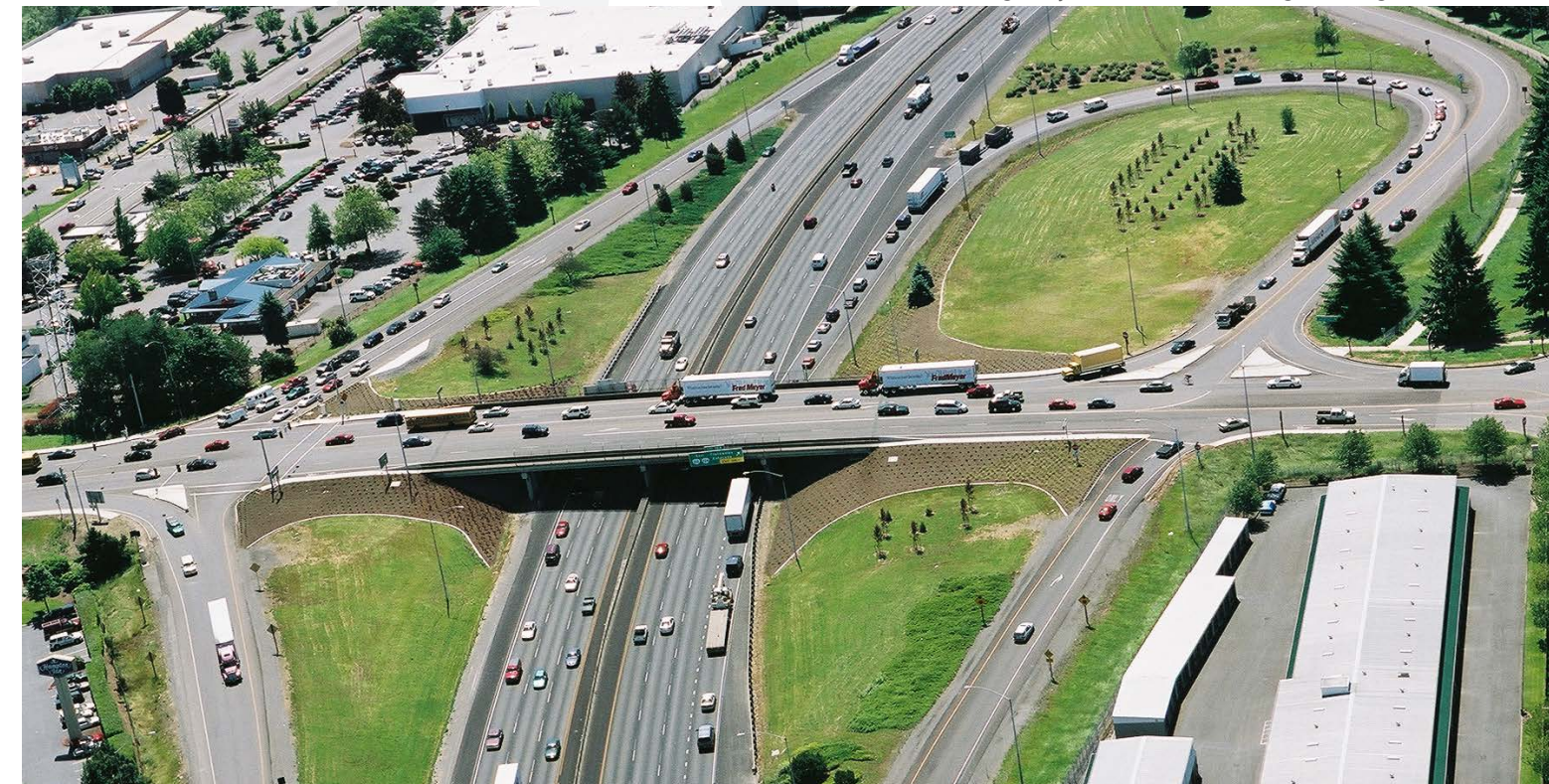
Highway 212/I-205 Interchange looking south
