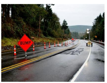
Cracks and southbound lane sinking below northbound lanes along OR 213 near Mulino.
