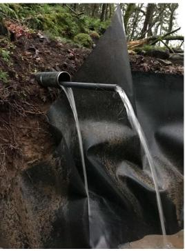
Drains inserted in the slope reduce additional slide movement.
