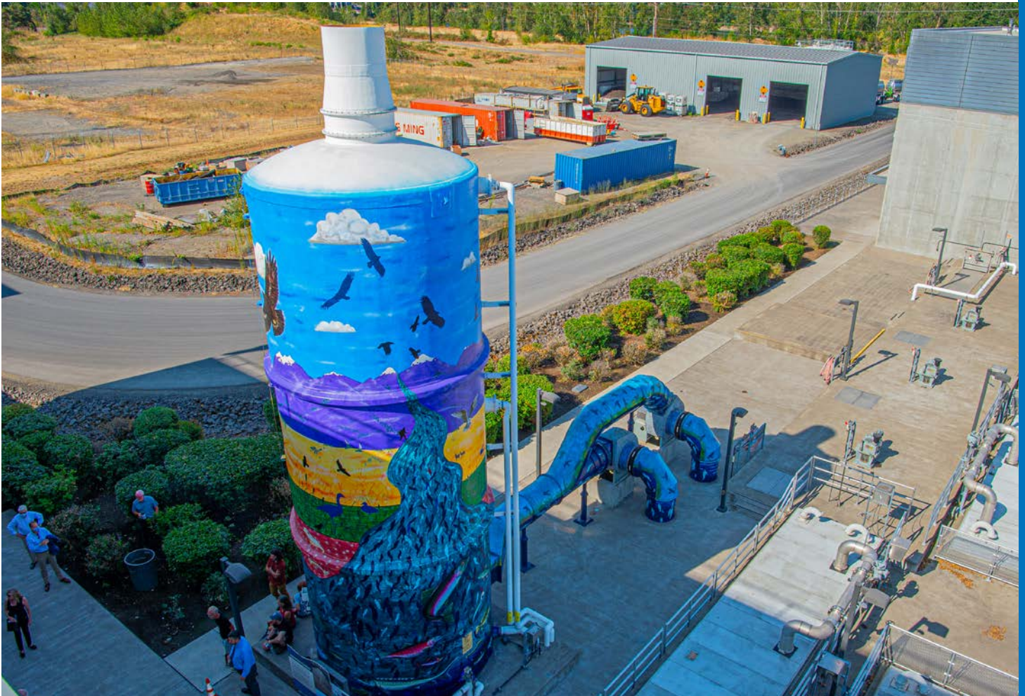
The new watershed health education mural on the odor control tower at the Tri-City Water Resource Recovery Facility
