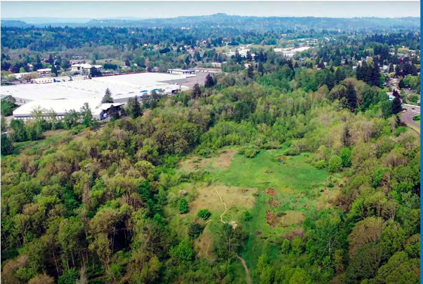
An aerial view of the 3-Creeks Natural Area Floodplain Enhancement Project
