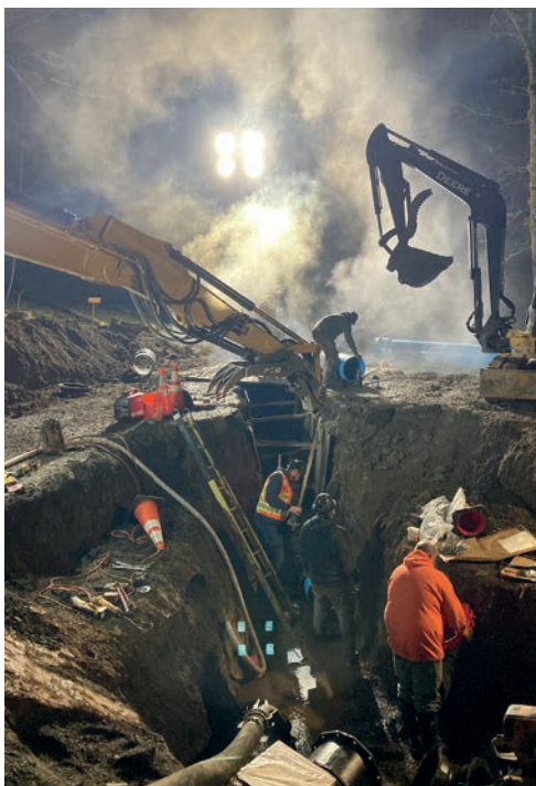
WES crews recently responded to a failing pipe in the Maddax Woods area of West Linn and conducted overnight repairs while preventing service interruptions.
