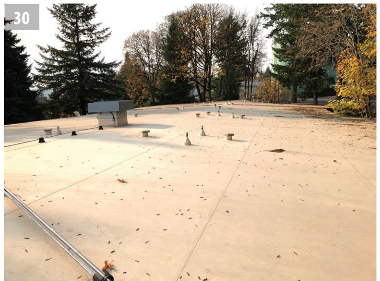
TPO roof over the west wing.
