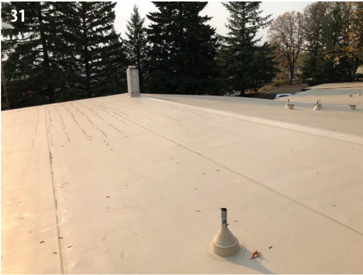
TPO roof over the center area.
