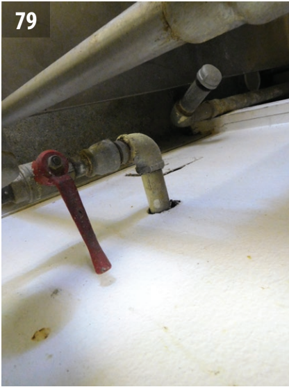
Galvanized-steel piping at the kitchen.
