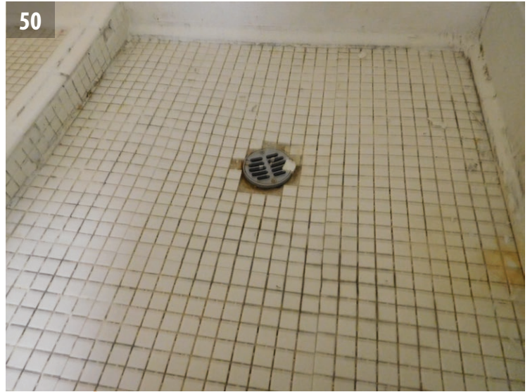
Floor tile in the shower room at the west wing.
