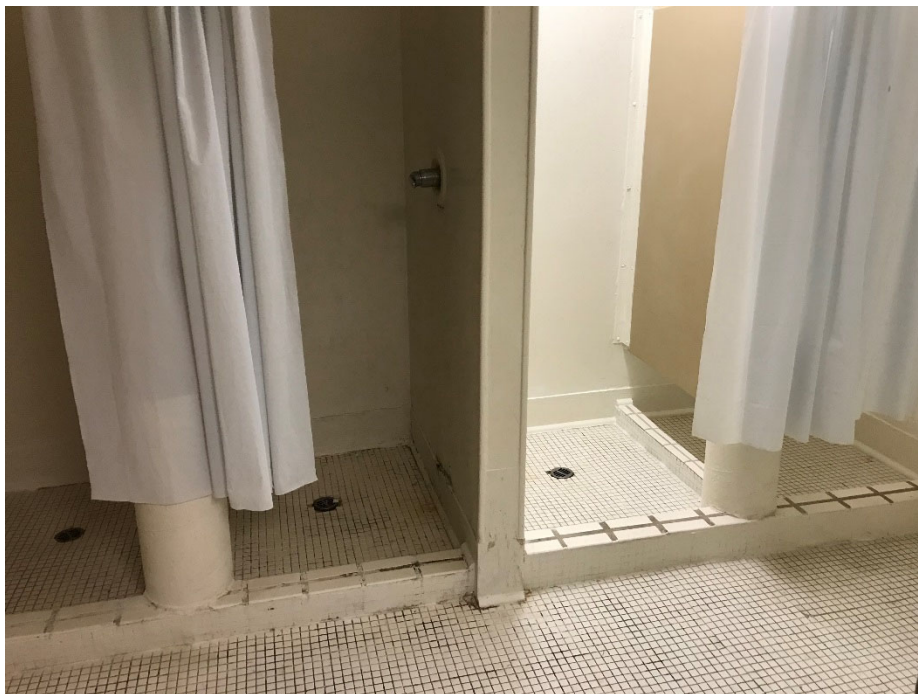
Photo 4. Typical shower room
