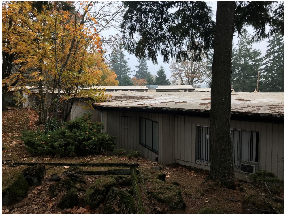
Photo 16. Northwest corner of the site, looking east
