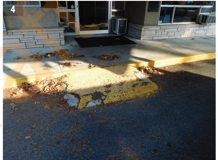
One of two asphalt curb ramps near the front entrance.
