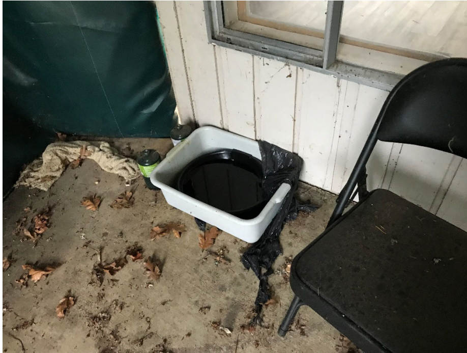
Photo 7. Oil pan with used oil outside eastern wing exit
