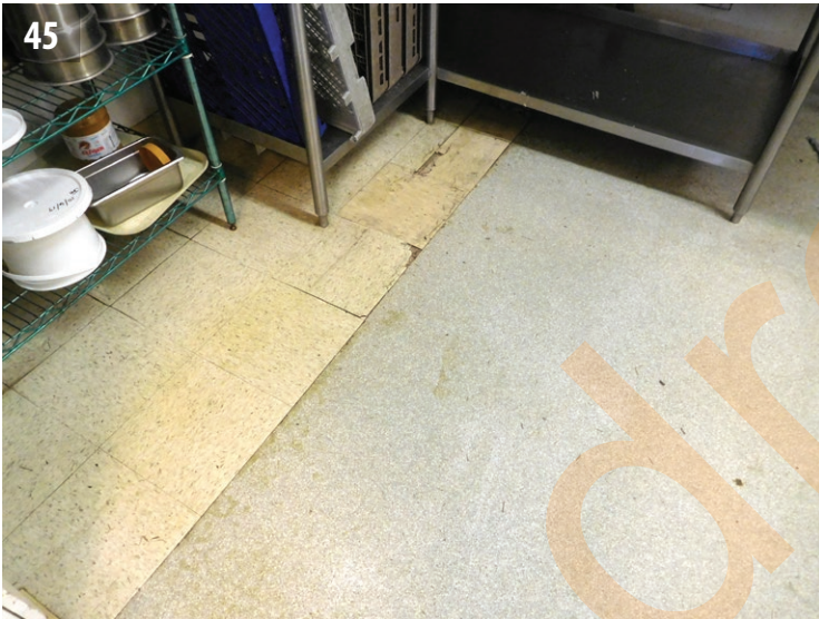
Section of VCT flooring in the kitchen.
