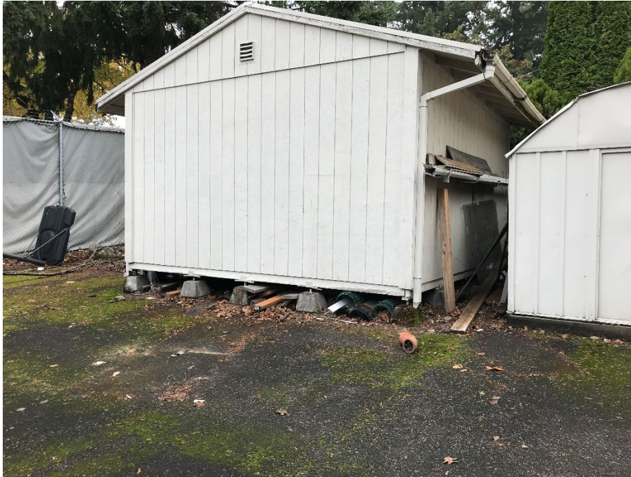
Photo 11. Maintenance building (used to store equipment and parts for building repair)
