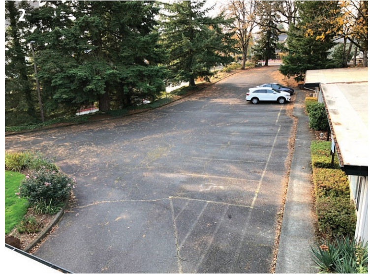
Asphalt drive and parking area, looking west.
