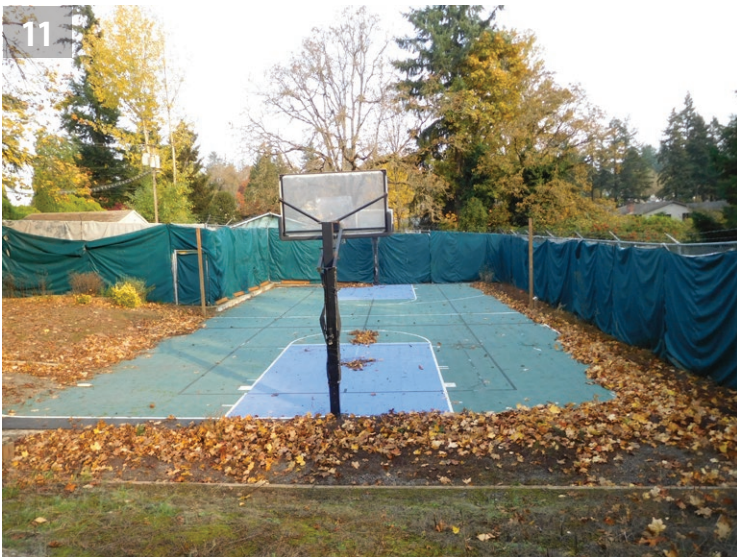
Sport court and fence at the rear of the property.
