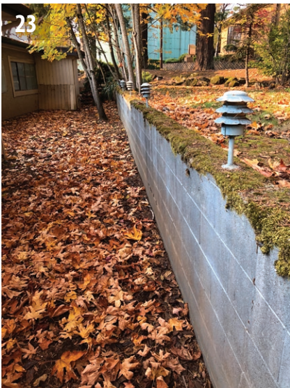
Retaining wall along the west side of the site.
