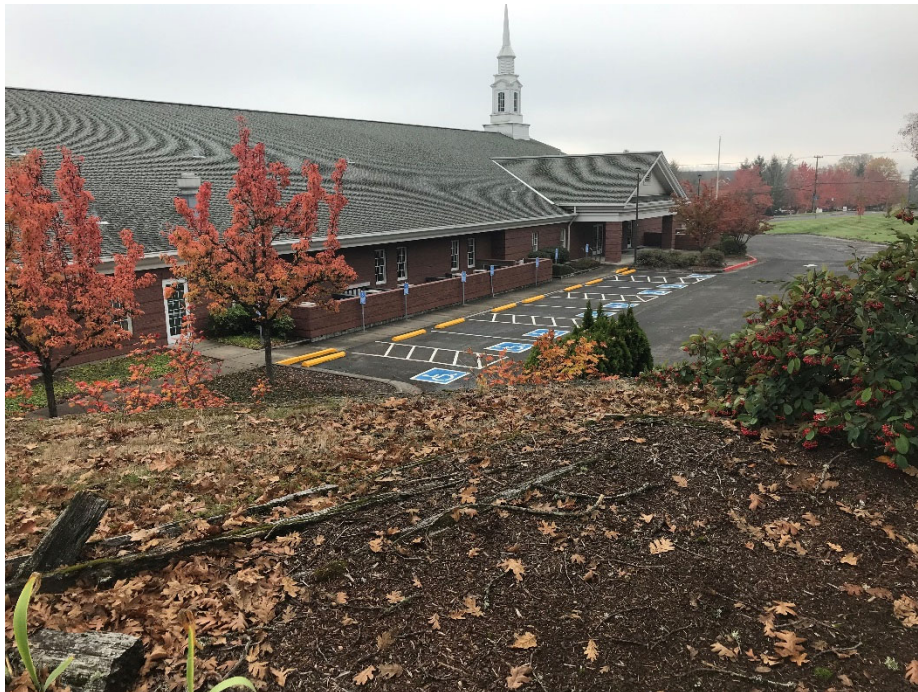
Photo 20. Southern adjacent property
