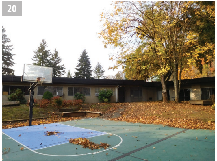
Rear elevation and sport court.
