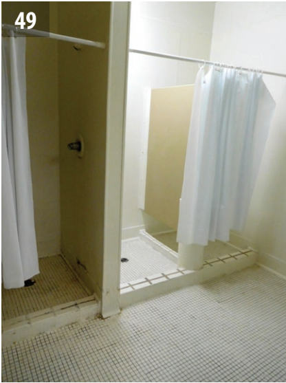
Shower room at the west wing.
