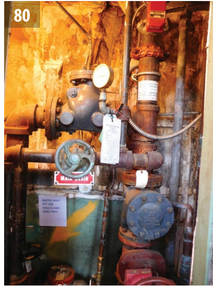
Fire-protection-sprinkler riser.
