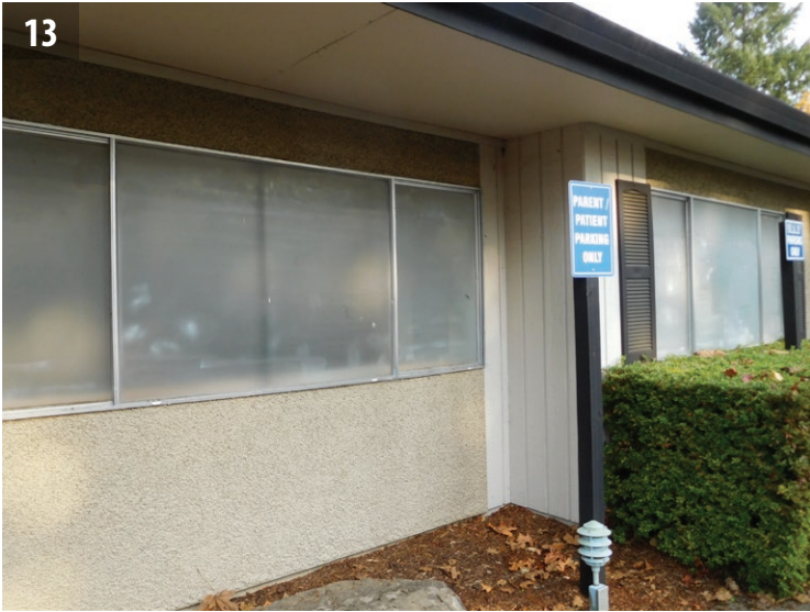
Aggregate-faced panels and aluminum-framed windows at the south elevation of the west wing.
