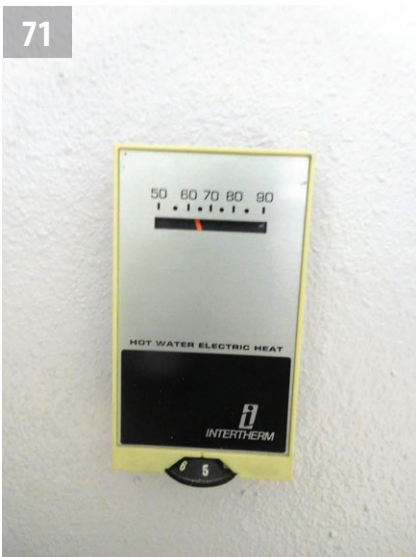
Intertherm thermostat for a hot-water electric heat baseboard radiator.
