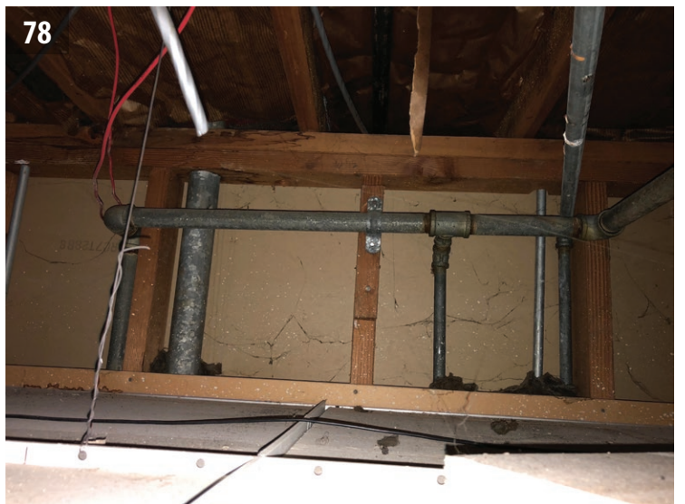
78 Galvanized-steel domestic-water piping and waste stack observed above the corridor ceiling.
