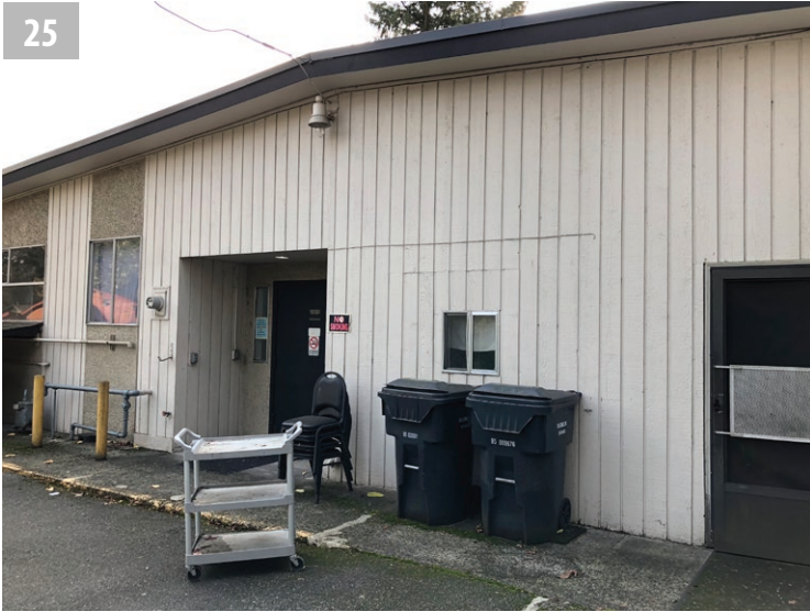
North elevation at the north wing.
