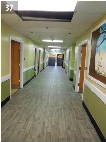
Common corridor at the north wing.
