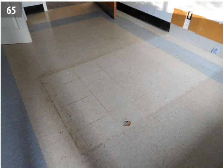
65 VCT flooring at Unit 26.
