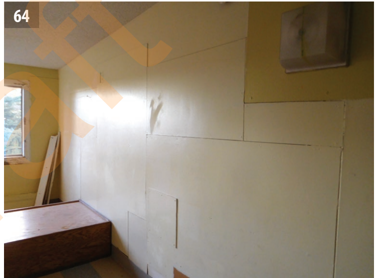
64 Walls patched with sheathing in lieu of GWB at Unit 25.
