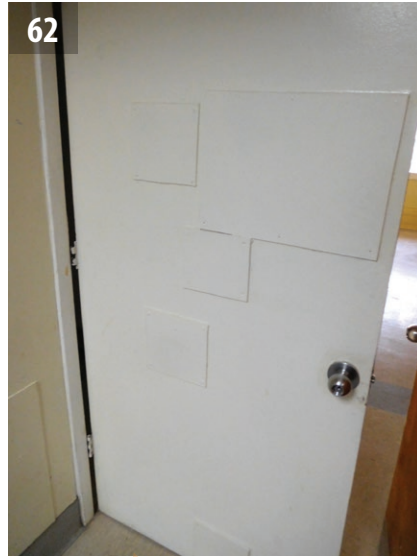
62 Patched bathroom door at Unit 22.
