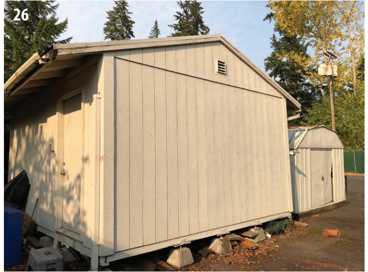
Maintenance and storage sheds at the rear of the site.
