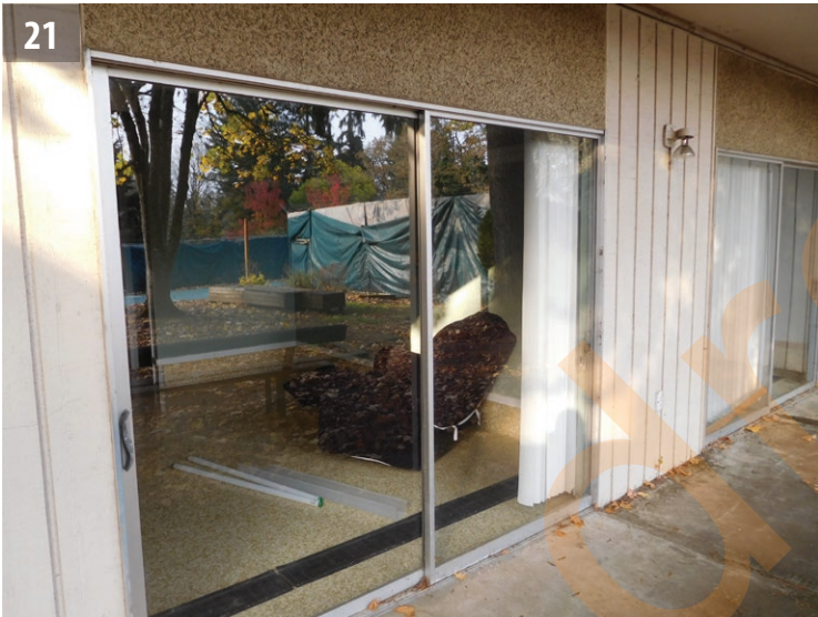
Aluminum-framed, sliding-glass door at the rear elevation.
