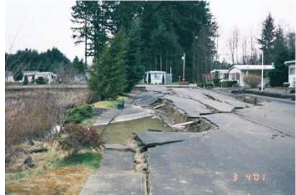
Image 18: Image of lateral spreading due to liquefaction in Tumwater, WA (Photo from USGS website & Geomatrix)
