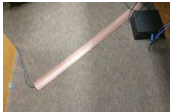
Image 3: Cables at litigation well in Courtroom
