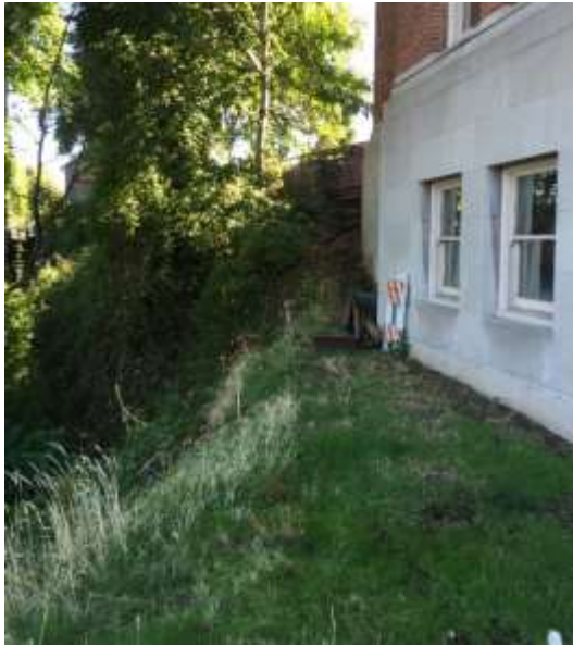
Image 17: Cliff at Willamette River (looking north)
