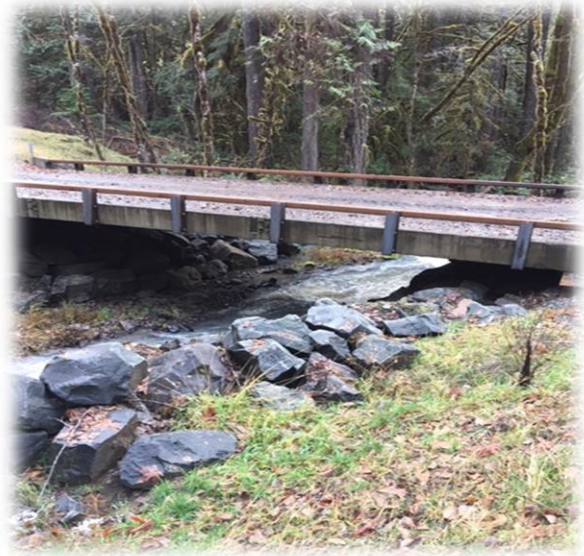
Smith Creek Restoration Project.
