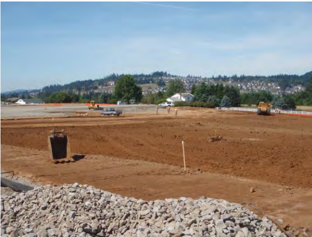
Photo 1-7. New development in the RC watershed
