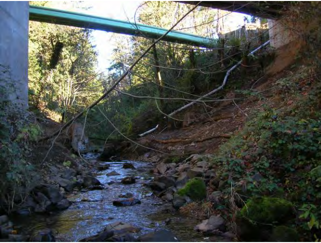
Photo 1-2. Rock Creek at Highway 224 bridge
