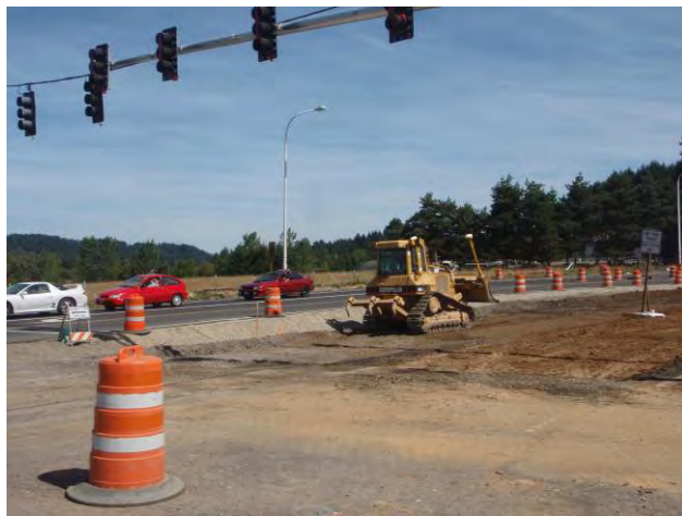
Photo ES-8. Road expansion in the RC watershed
