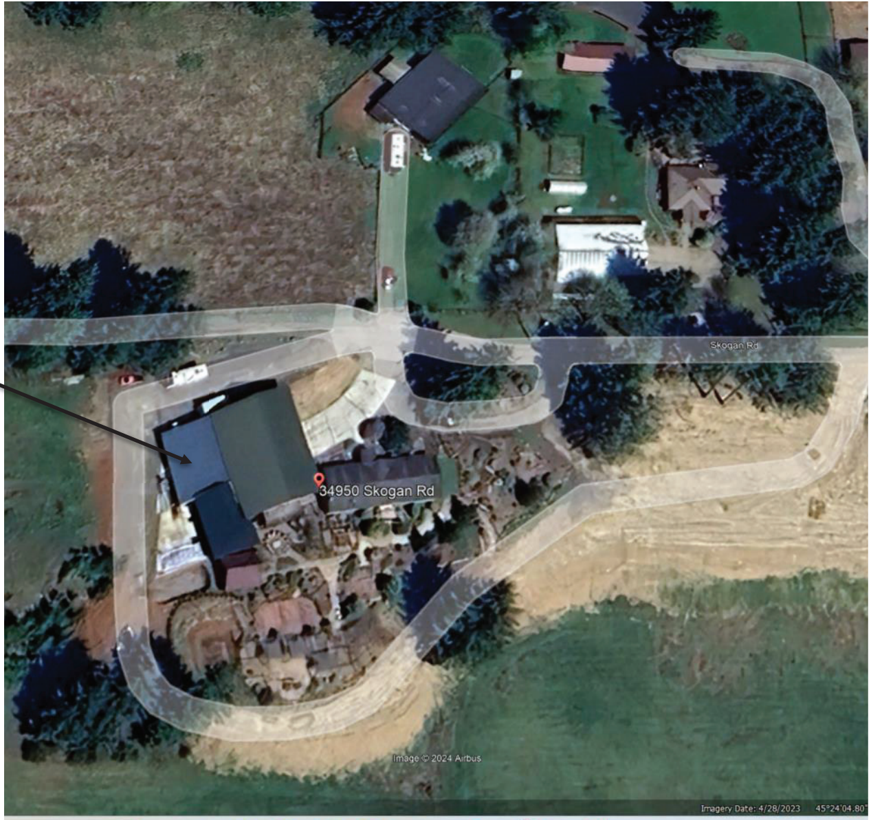
Aerial – 4-28-2023 – Another addition to the structure
