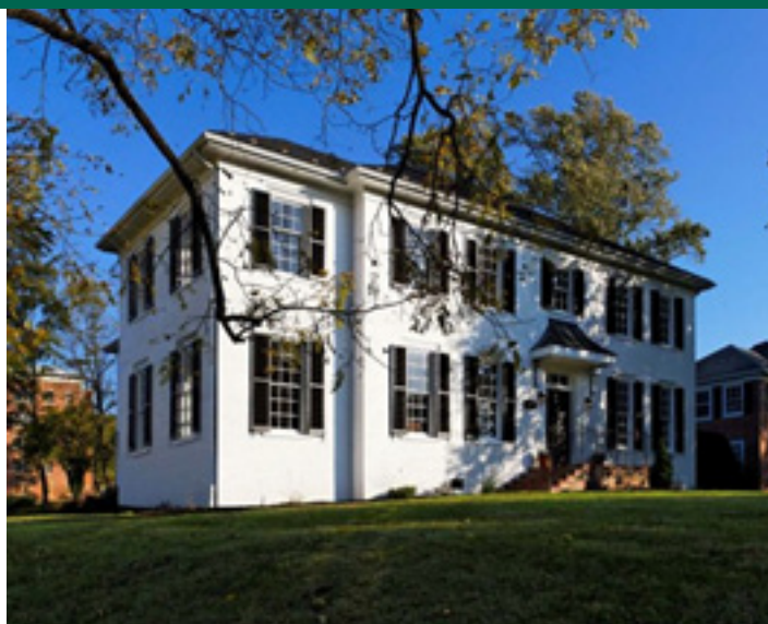
Residential property in Staunton, Virginia, rehabilitated using Virginia state historic preservation tax credits. Source: Miller & Associates, http://www.robinmillerassociates.com/historic-tax-credit .
