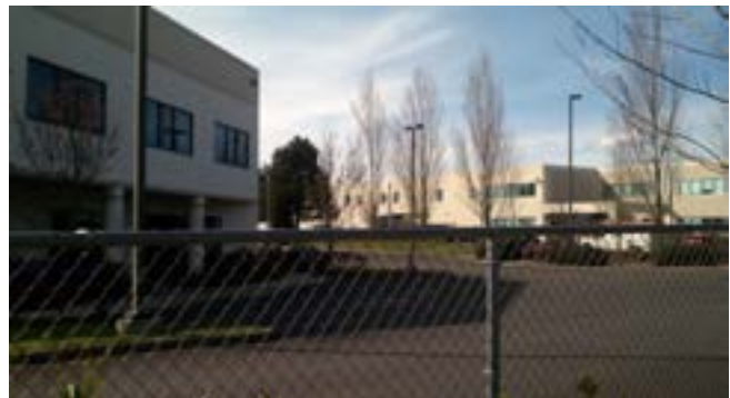
Existing chain link fencing at Silver Oak easement Fence: chain link, 4-foot high.
