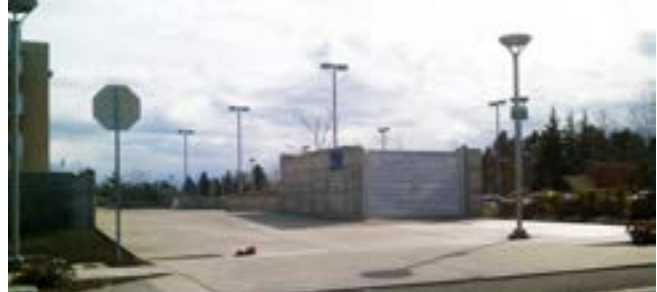
Louvered fence at DSB transformer, Library Court Fence: Concrete and louvered metal panel, 12-foot high. Concrete and Mealt pane
