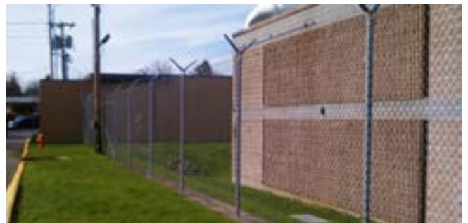
Existing perimeter fence at ADF Fence: Chain link with barbed wire, 8-foot high.
