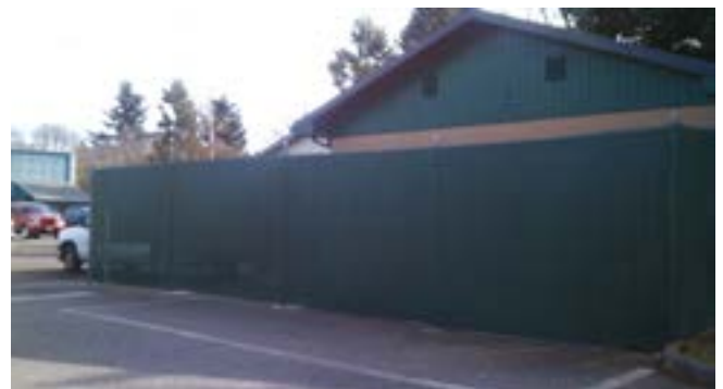
Existing screening at Sheriff's Facility Fence: Slatted chain link, 8-foot high.
