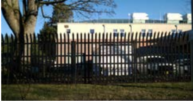
Portland Dispatch Center's Forked Privacy Fence Painted metal with forked top, 8-foot high.
