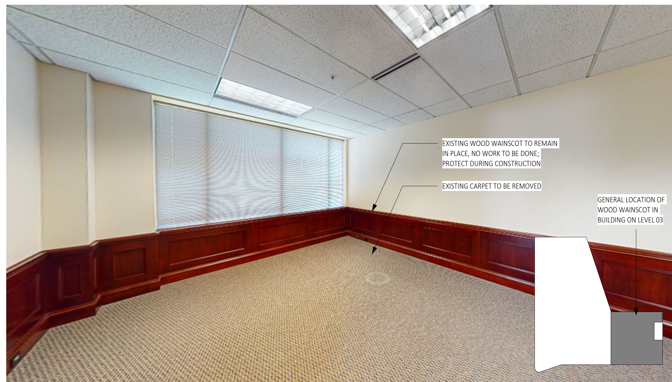
EXISTING WALL PANELING ON LEVEL 03 (Q&D TRAINING ROOM)
