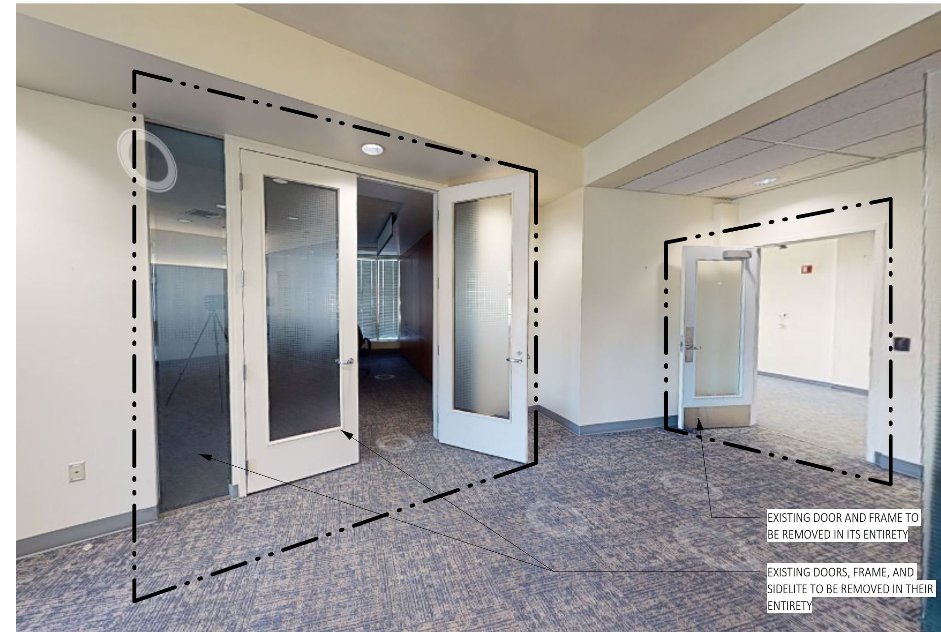
EXISTING LOBBY ON LEVEL 02 (LOBBY 201)
