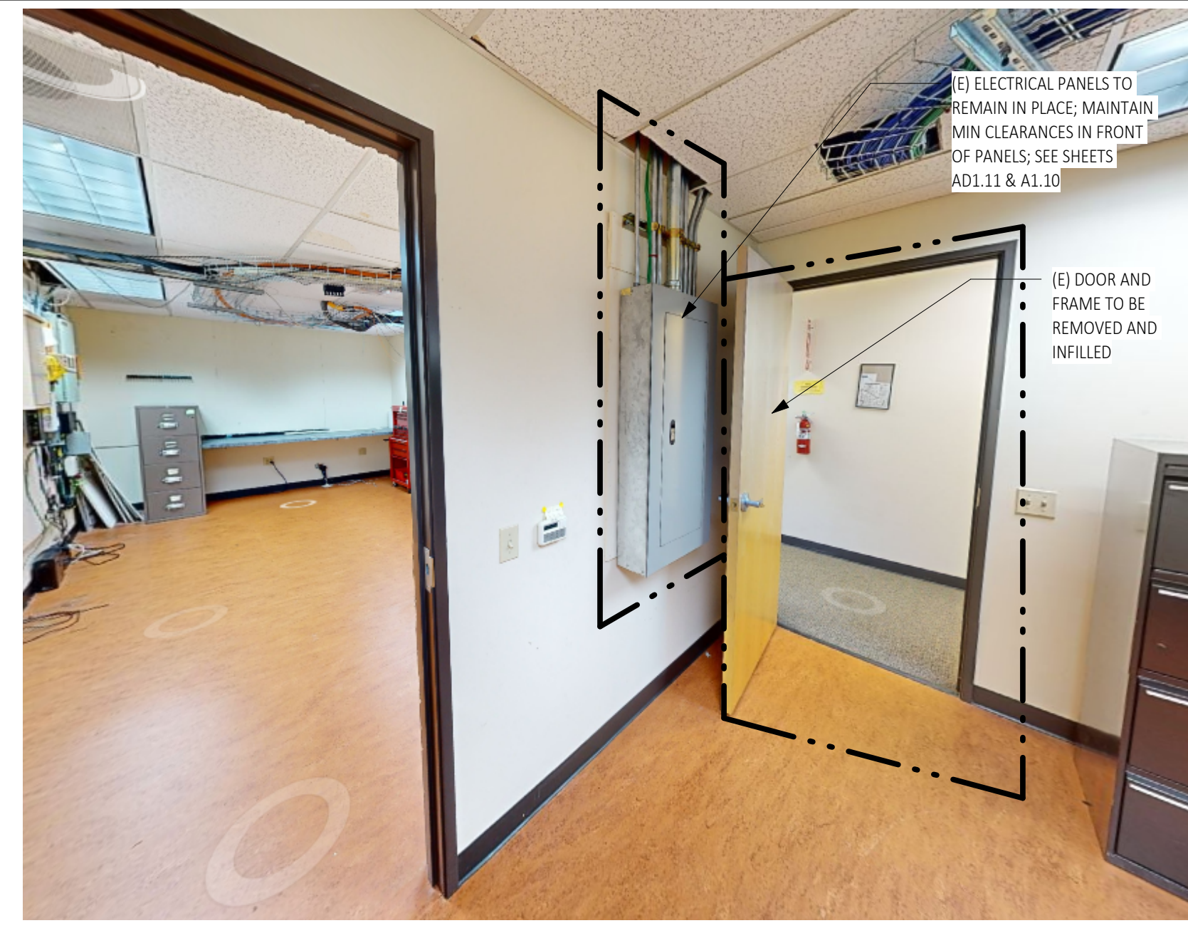
EXISTING ELECTRICAL ON LEVEL 01 (IT 122)
