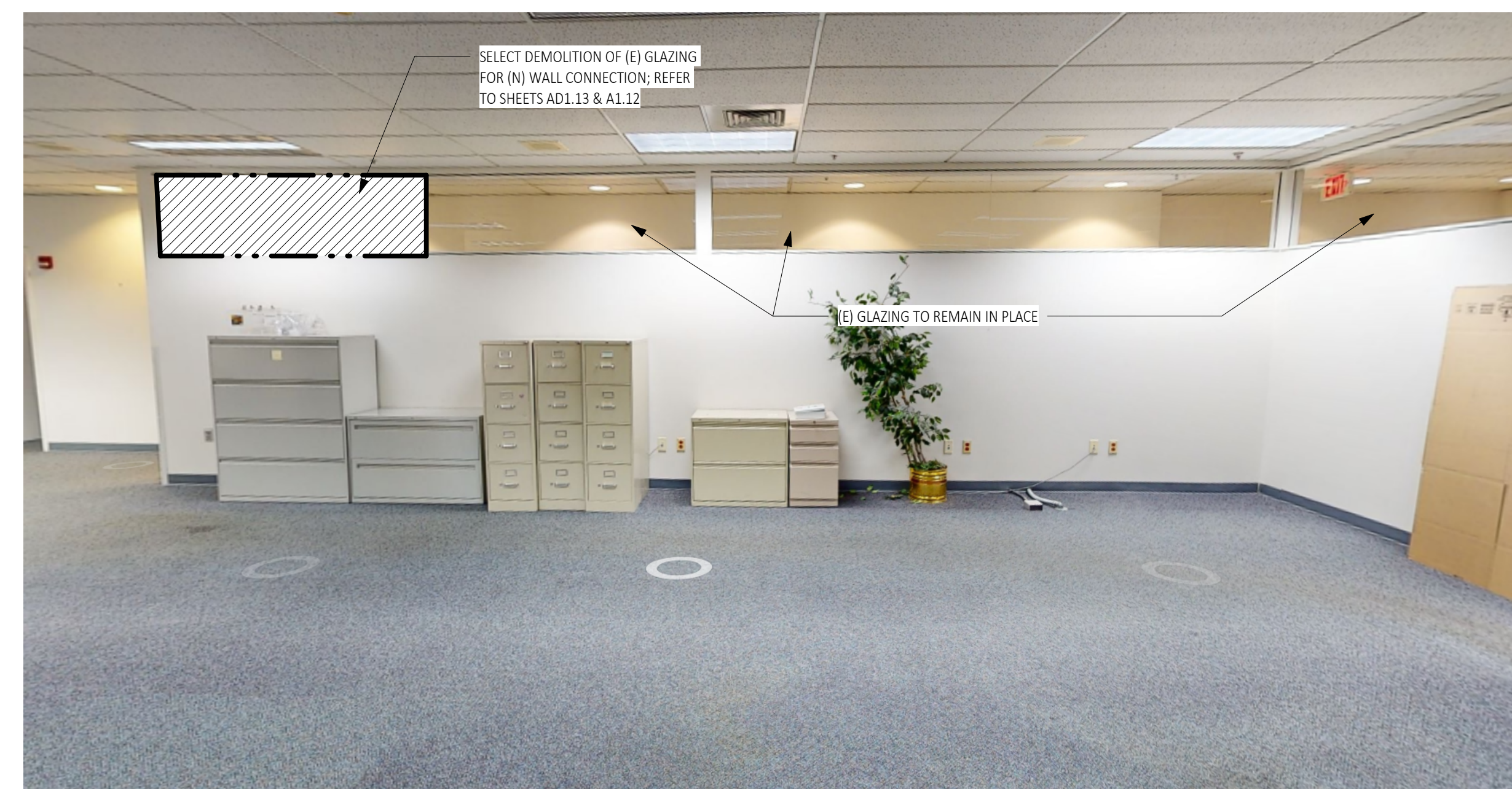
EXISTING CLERESTORY GLAZING ON LEVEL 03 (GROUP ROOM 324)
