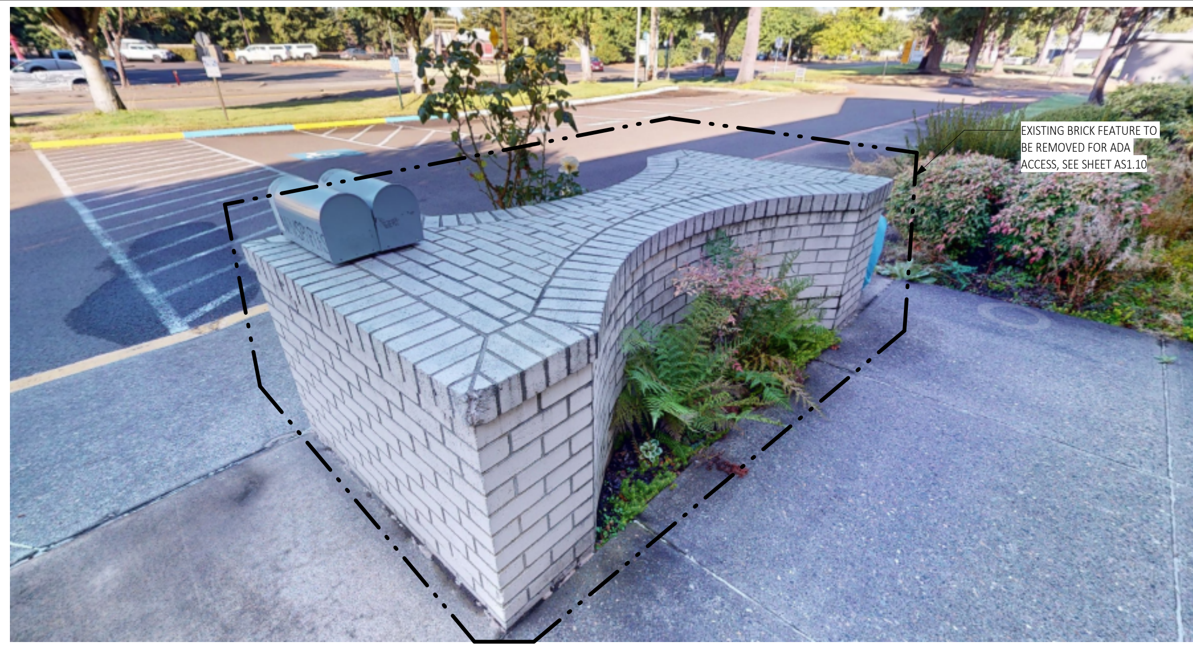
EXISTING BRICK AT BUILDING ENTRANCE
