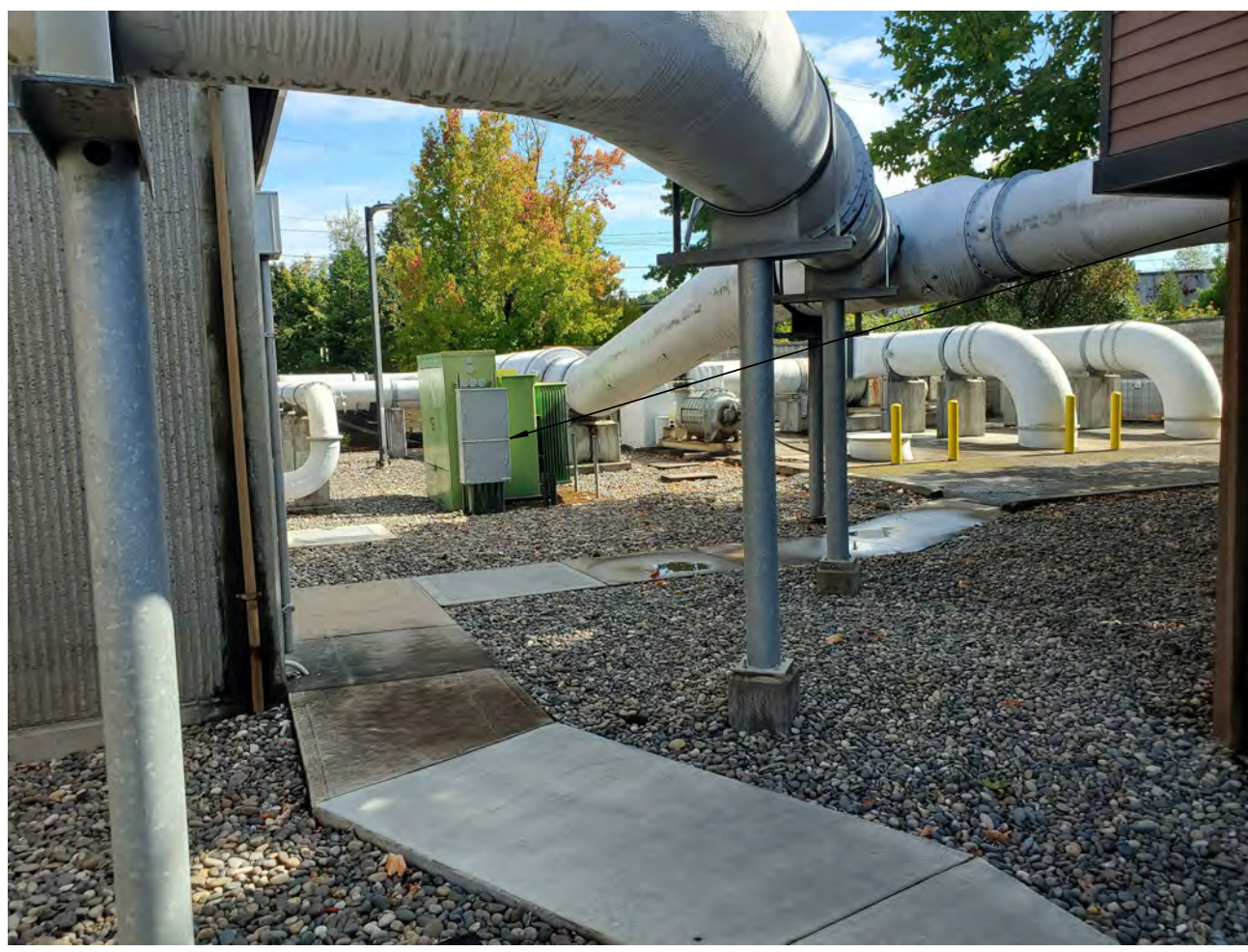
B PHOTOGRAPH 12 - ABANDONED 1000 KVA TRANSFORMER NO SCALE
