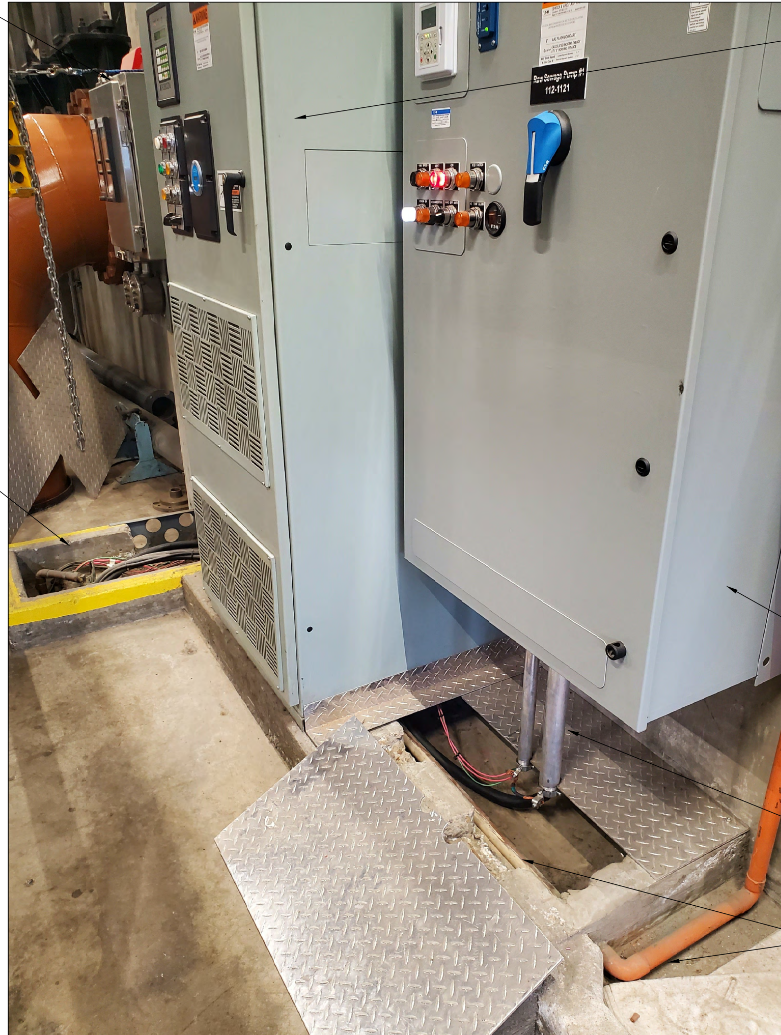
D PHOTOGRAPH 8 - PUMP 1 AND 2 VFD CABLE TRENCH E-103 NO SCALE
