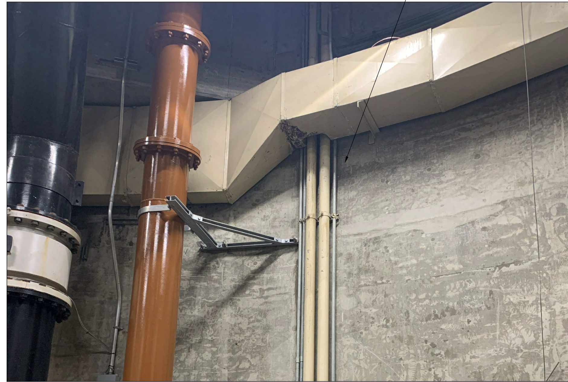
A PHOTOGRAPH 9 - EXISTING PUMP CONDUIT (MOTOR LEVEL) E-101 NO SCALE
